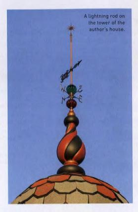
at intervals along high points such as the roof crest, ridge, chimney, or along the perimeter of a flat roof. A braided copper or aluminum cable made for lightning systems connects the rods and runs into the ground to dissipate a charge. To avoid oxidation and even fire, don't mix copper and aluminum components; thus, don't use a copper rod with aluminum roofing or siding. Keep aluminum components away from copper roofing or gutters.
