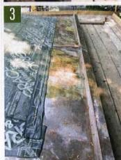
Closeup of sistering stabilization measures, with steel straps installed under the gutter. 3. View of gutters and substrate fully covered by the ice and water membrane. 4. A view of the finished roof.
