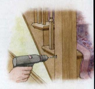
bit that matches the size of the fastener head; go just deep enough to countersink. Using a long drill bit the same diameter as the screw, drill through the side of the post into the edge of the tread, keeping the drill level. Cover the hole with wood putty; finish to match.
