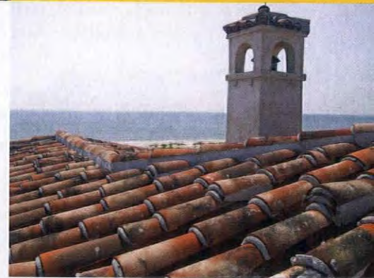
TOP Concrete roof tiles like these from Bartile come with detailed installation instructions and can be ordered with standard installation materials such as eave risers and proprietary ridge vent systems. ABOVE Mission (or barrel) tile is one of the oldest forms of roof tile, originally formed over the thighs of workers. The tiles in this barrel-tile roof were made by Ludowici Roof Tile.
