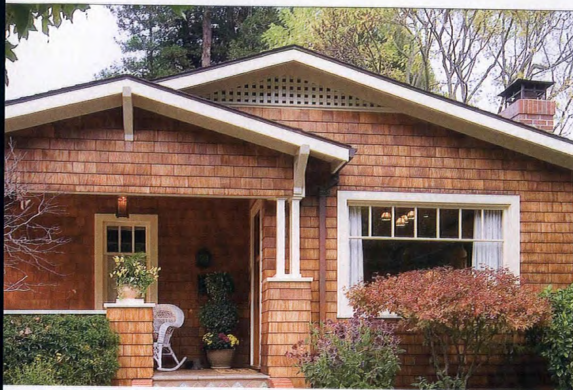
LEFT This lattice-work gable vent in a restored bungalow is a variation on historic attic vents that were common a century ago. If necessary, add additional ventilation along the soffits, the lowest point on the roof.
