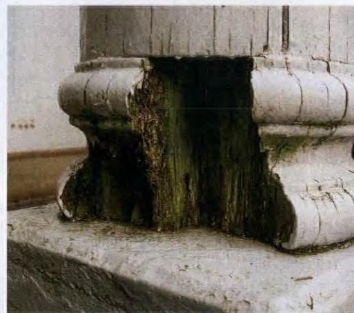
ABOVE An unvented wood column eventually rots from the inside.
