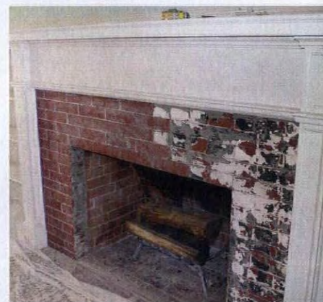
ABOVE Never paint a brick or stone surround—or a future owner may be forced to do this. LEFT Blue Bear's Soy-Gel removes paint from masonry safely and easily.
