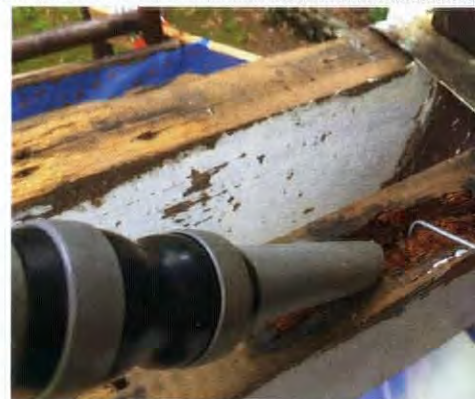
ABOVE Damaged wood in the decay zone is scraped with a mechanic’s pick as a HEPA vacuum keeps things clear.
