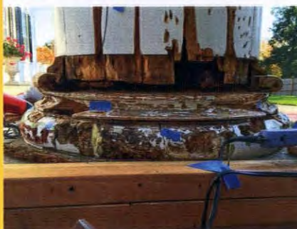
Repair of exterior columns using ConSolv Epoxy products involved liquid borate preservative, epoxy consolidation, epoxy filling and shaping, and new wood at the base.
