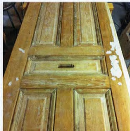
CLOCKWISE FROM LEFT The antique maple door required sanding, stripping, and repairs. • Never reach into the second tub of epoxy with the same gloved hand. • Epoxy-filled voids left by old hardware and hinges. • The door frame after curing and sanding.
