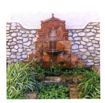
Combining mixed materials of varying size and thickness requires a skilled tile installer. The mortar bed must be manipulated to assure a **level surface**, and grout **lines adjusted** for looks.
