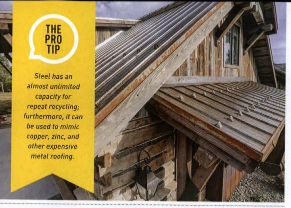
rusty appearance of Bridger Steel's Truten® weathering steel actually protects the steel inner core. especially popular in the West.
