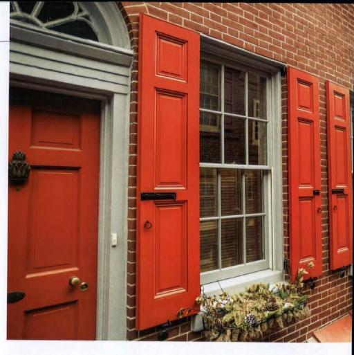
tion. The best are built using mortise-andtenon construction.
