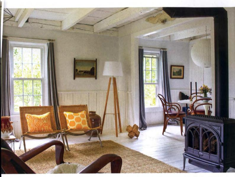
**ABOVE** In main rooms, acoustical tile and mid-19th-century plaster ceilings were removed to reveal the hand-hewn beams. Original wide-plank floors are pine.
