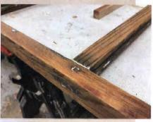
ABOVE RIGHT The sash is lavishly coated in a 50/50 mix of boiled linseed oil and turpentine. The turpentine allows the oil to penetrate old, damaged wood, then evaporates as the oil cures. BOTTOM After three coats of BLOP were fully cured, the author hand-sanded the sash with 400-grit sandpaper.
