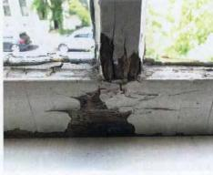
**Stripped to Perfection** Stripping is undoubtedly the most tedious part of window restoration. Old school, less-than-ideal methods like dipping the sash in **toxic solvents or using a heat gun on the old, fragile wood (near glass) have been superseded by gentler techniques** that harm neither wood nor glass, including infrared heat
