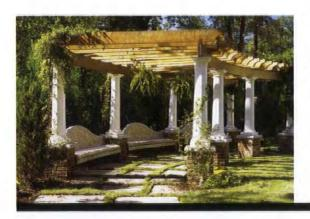
TOP Western red cedar is naturally decay resistant and less expensive than tropical woods, making it a good alternative to pressure-treated lumber for some uses. LEFT Chadsworth's architecturally correct Polystone columns—made of fiberglass, resin, and marble dust—are stronger than wood and last longer in areas exposed to water.
