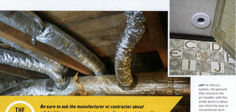
winterizing a new mini-duct system. If you do not close off the ceiling ducts and attic returns, moisture will accumulate in the system and may cause damage as well as mold issues. ing. ABOVE Mini-duct outlets are small and may be ordered in colors that match the ceiling or wall.
