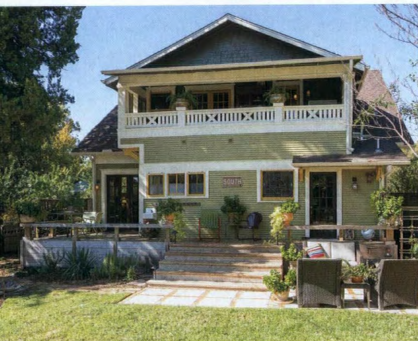
ABOVE The removal of a rusted screen porch and addition of a period balustrade enhanced the rear façade. These owners added a patio of concrete blocks and salvaged bricks. RIGHT The half-timbering in the gable had been removed; the landmarks commission agreed to its reinstatement once the connection to Wilson design No. 492 was established.
