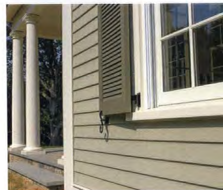
TOP Fiber-cement siding from James Hardie's Aspyre collection is \frac{5}{8} " thick and casts realistic, deep shadow lines. MIDDLE Ecoshel's pre-assembled cedar-shingle systems are marked for optimal spacing and install five times faster than individuals. ABOVE GAF reproduces three patterns of Fifties-style shingles in fiber cement. BELOW The clapboards are rot-resistant Western red cedar.
