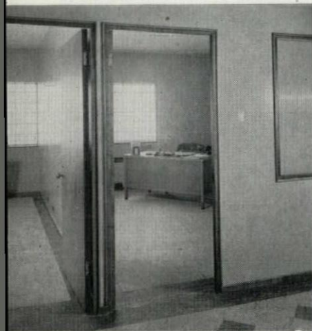
Above, left, U. S. Gypsum's 2"-thick partition construction; right, thin precast concrete wall with prestressed reinforcing, lifted into place by vacuum beams, Vacuum Concrete, Inc. Below, 130-ft. span continuous reinforced concrete rigid frames, precast joists and slabs, roof a flight hangar
