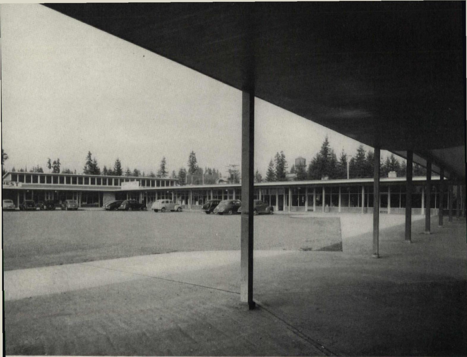
Sound principles for postwar planning—stores planned as a unit; car parking adjacent, shelter from sun and rain; simple materials, simply used
