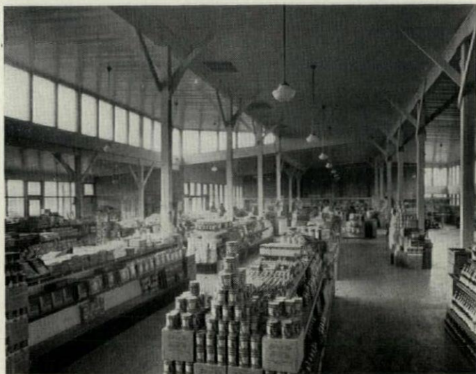
Both wall windows and clerestory daylight the market
