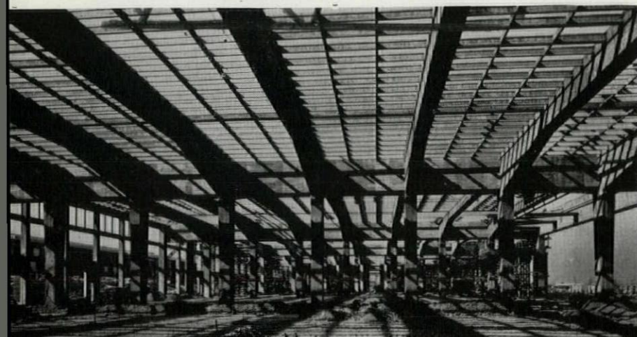
Above, left, U. S. Gypsum's 2"-thick partition construction; right, thin precast concrete wall with prestressed reinforcing, lifted into place by vacuum beams, Vacuum Concrete, Inc. Below, 130-ft. span continuous reinforced concrete rigid frames, precast joists and slabs, roof a flight hangar
