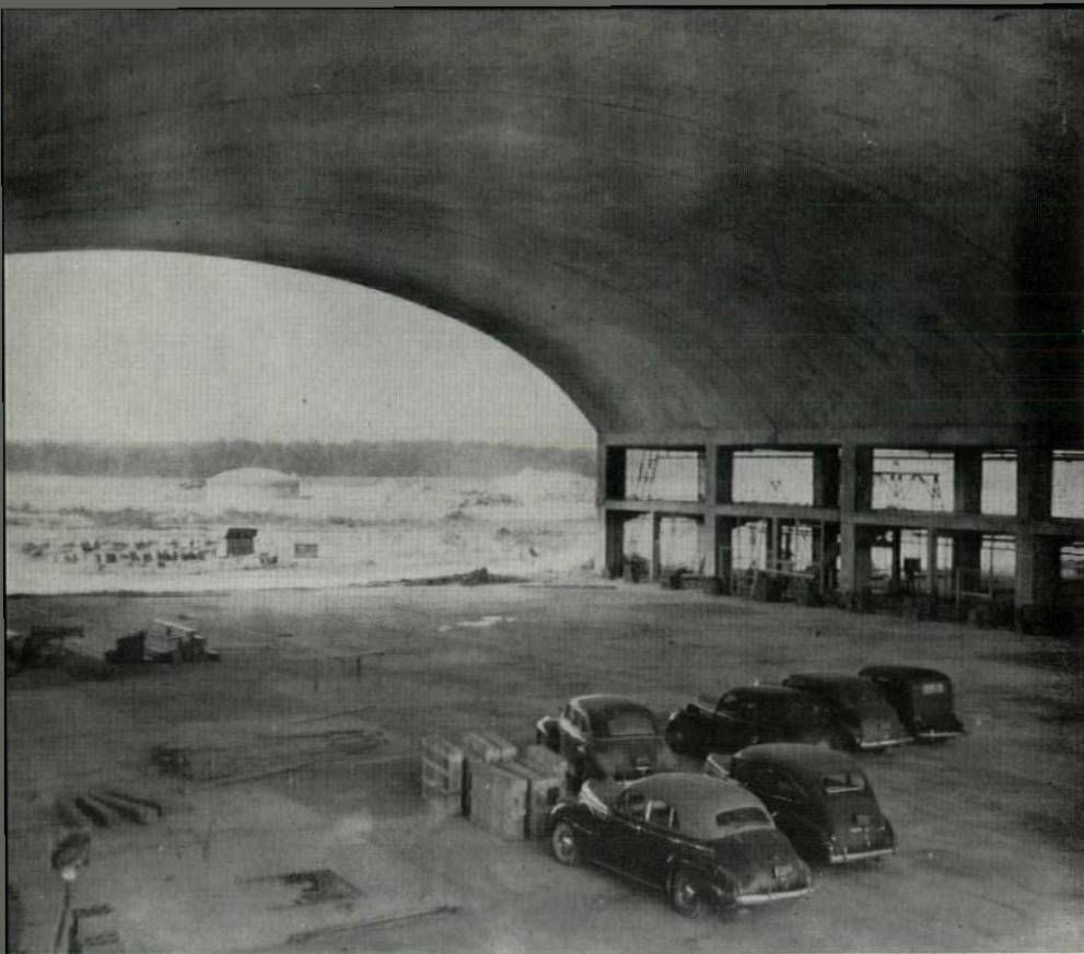
Above, navy hangar, a thin-shell arch in concrete, span 160 ft., shows effect of airplane development in helping to popularize this type of construction
