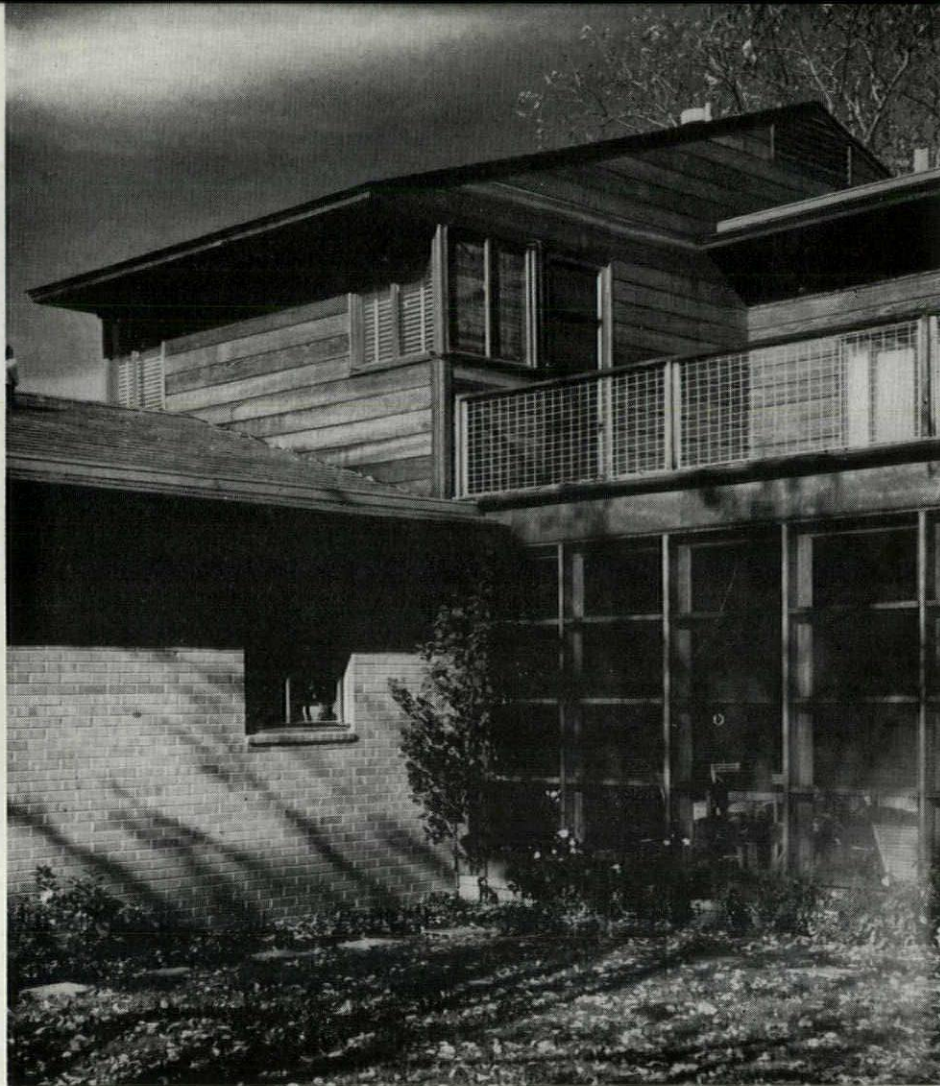
The garage wing (left) and house proper shield the living porch and garden from street view and noise. Construction is of wood frame, built on reinforced concrete piers and grade beams. Brick veneer surfaces the ground floor. Above, V-joint redwood shiplap is used. The roofing is black slate
