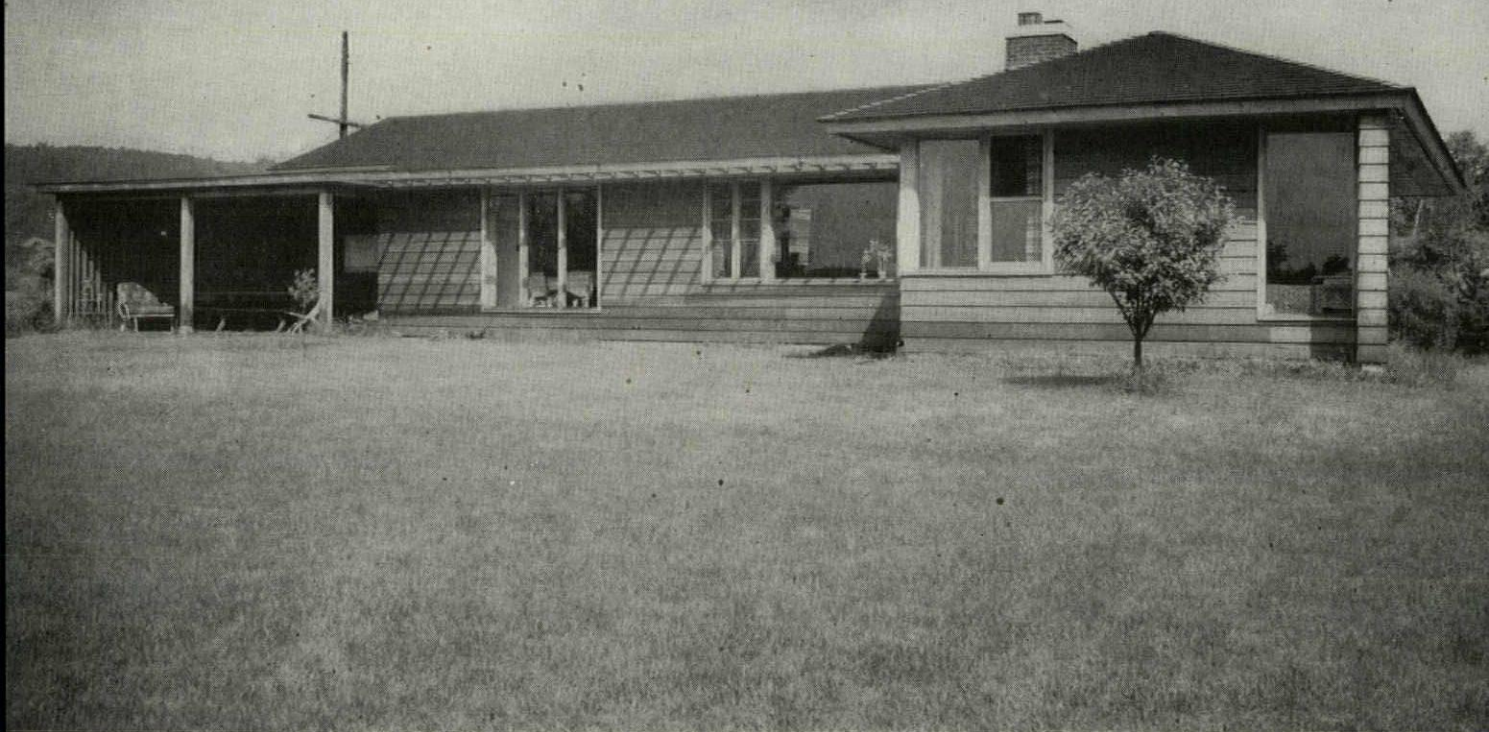
Southern front, showing large window areas and projecting eaves that control amount of sunlight
