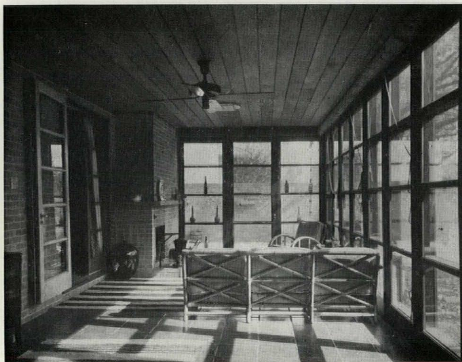
The living porch. During the winter, the porch is enclosed with glazed panels that in summer are stored in special closets in the garage
