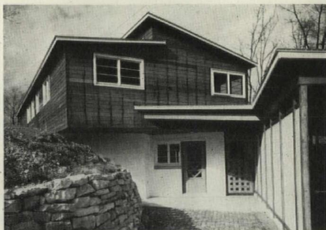
Main entrance, service entrance, and carport are concentrated to open off the main roadway level
