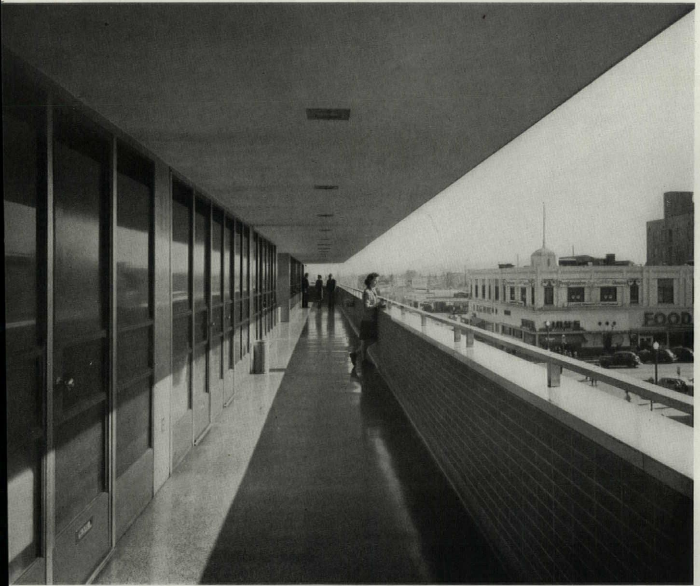
A cantilevered sidewalk around the south and east sides of each office floor replaces the usual interior corridor and provides shade for the office wall below. East and south walls consist of metal-framed panels of obscure glass. All photos were taken about November 20 and show nearly maximum sun penetration.
