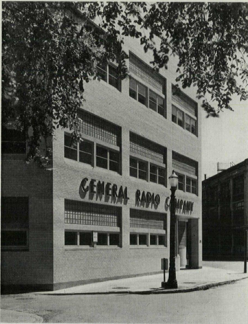
Panels of glass block control direct sunlight on southern and western walls; in the photograph below, a portion of the factory proper appears at far right
