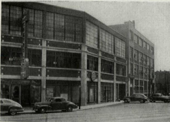
Before: old garage building
