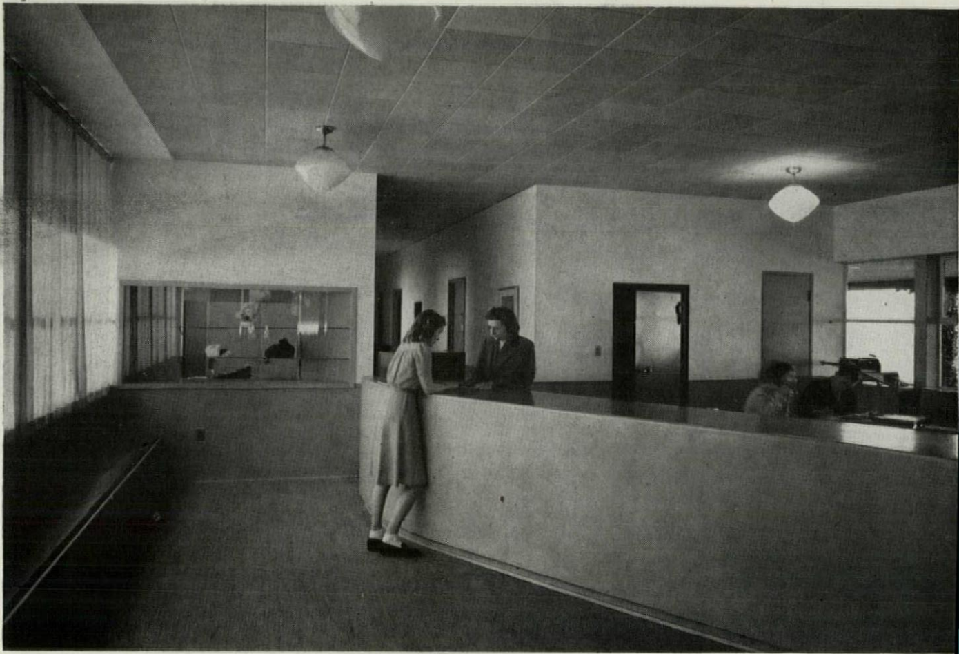
PLYWOOD-WAINSCOTED LOBBY OF ADMINISTRATION BUILDING; FLOORING IS LINOLEUM.
