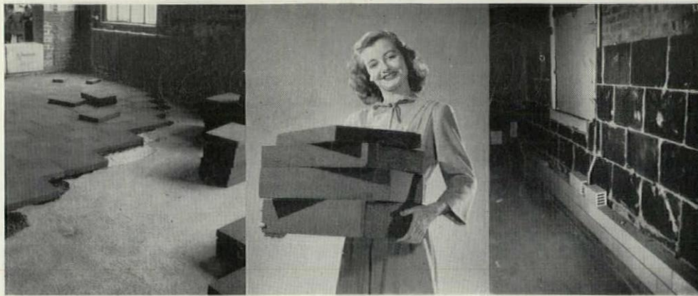
Cellular glass slabs, extremely light, designed for building into floors or roofs (left) or as cores of walls (right) to provide thermal insulation; photos courtesy Pittsburgh Plate Glass.
