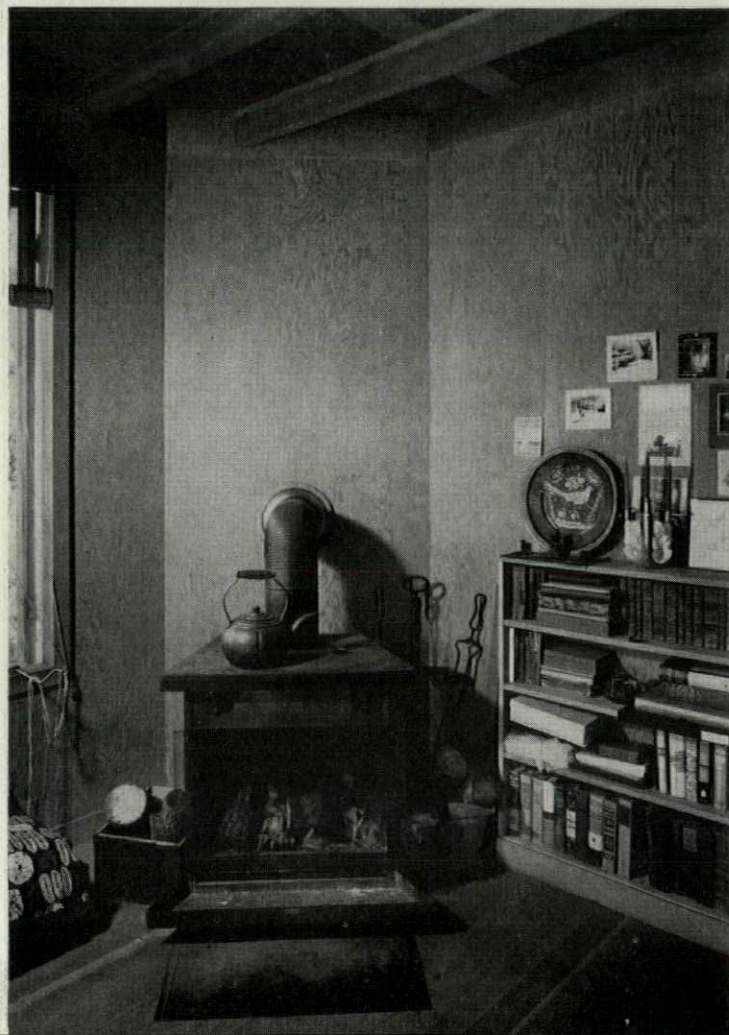
A Franklin stove heats the living room; walls are plain fir plywood sheets from floor to ceiling; flooring is T and G fir, finished with one coat of oil.
