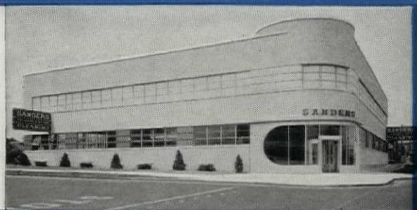
Truscon Pivoted Steel Windows in office, Pivoted Steel Windows in factory, and Open-Truss Steel Joists in Sanders Tri-Cleaning Co. plant, Detroit, Mich.
