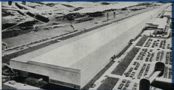
Truscon Ferrroglass construction in large southwestern bomber assembly plant.
