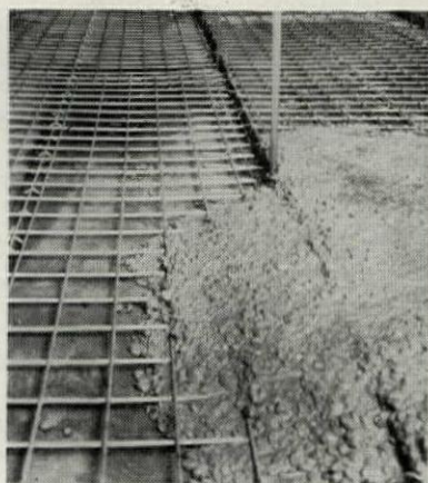
BEAM AND SLAB CONSTRUCTION. Welded Wire Fabric reinforces these ceiling slabs of the Smoke Chamber, Chicago Post Office, Chicago. Note the accuracy of placement and the rigidity of the Welded Wire Fabric Reinforcement.
