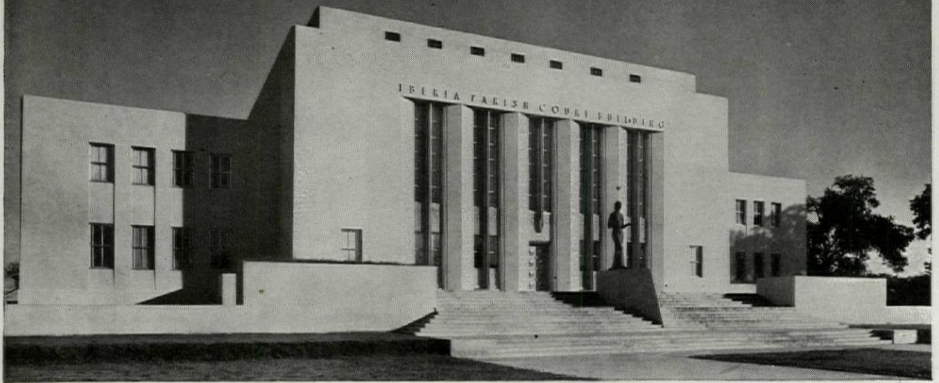
Iberia Parish Court Building in Louisiana is classical in form yet constructed of modern materials. It was designed in architectural concrete by Architect A. Hays Town of Baton Rouge. Engineer, Thomas Lucy, Baton Rouge. Contractors, Gravier & Harper, Lake Charles.
