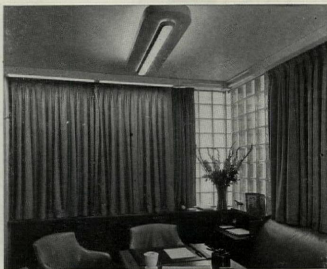
Study-type office or small conference room has lowered central fixture that provides both indirect general lighting and good working light on the desk itself.
