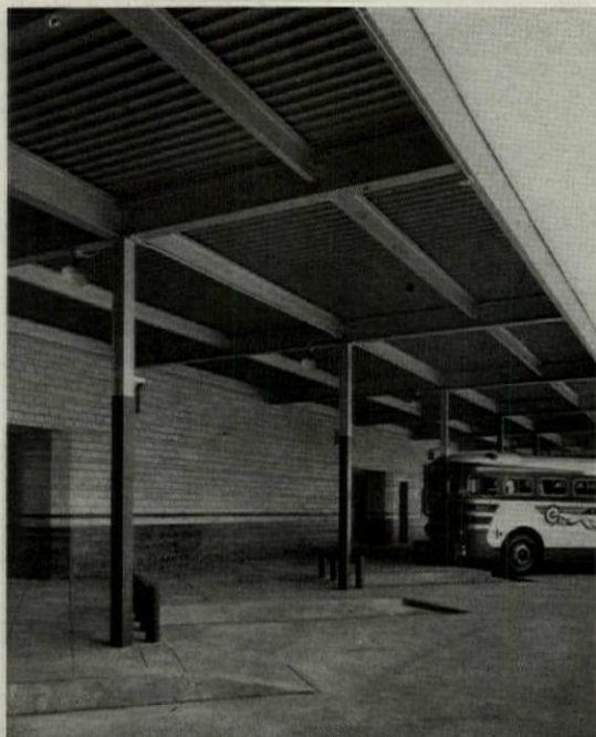
Detail of concourse.
