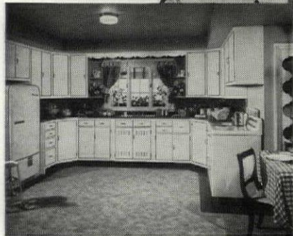
Curtis stock cabinets provide maximum convenience and storage space for any size or shape of kitchen.
