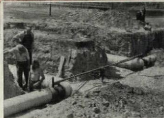
Ric-wil Prefabricated Expansion Loop "cold sprung" into position. Loops are fitted with drive couplers for easy assembly to straight runs.
