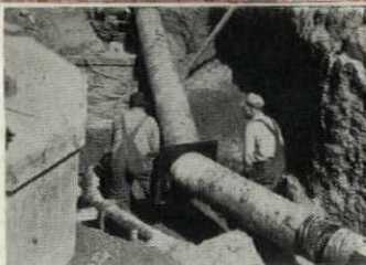
Installing Ric-wil Prefabricated Insulated Conduit on steam line to Firestone Laboratory. Note pipe and casing anchored at 45° offset.
