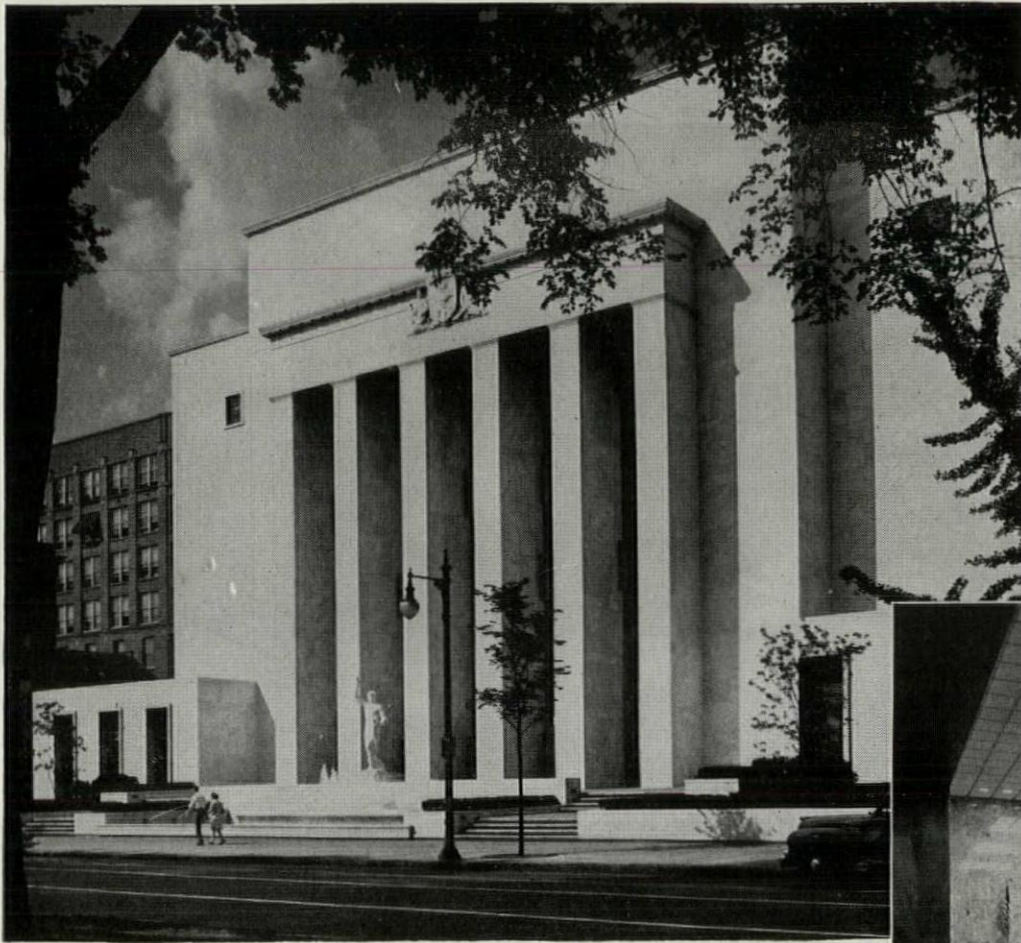
Dauphin County Court House, Harrisburg, Pa. Architects: Lawrie & Green, Harrisburg, Pa. General Contractor: Wm. A. Berbusse, Jr., Inc.
