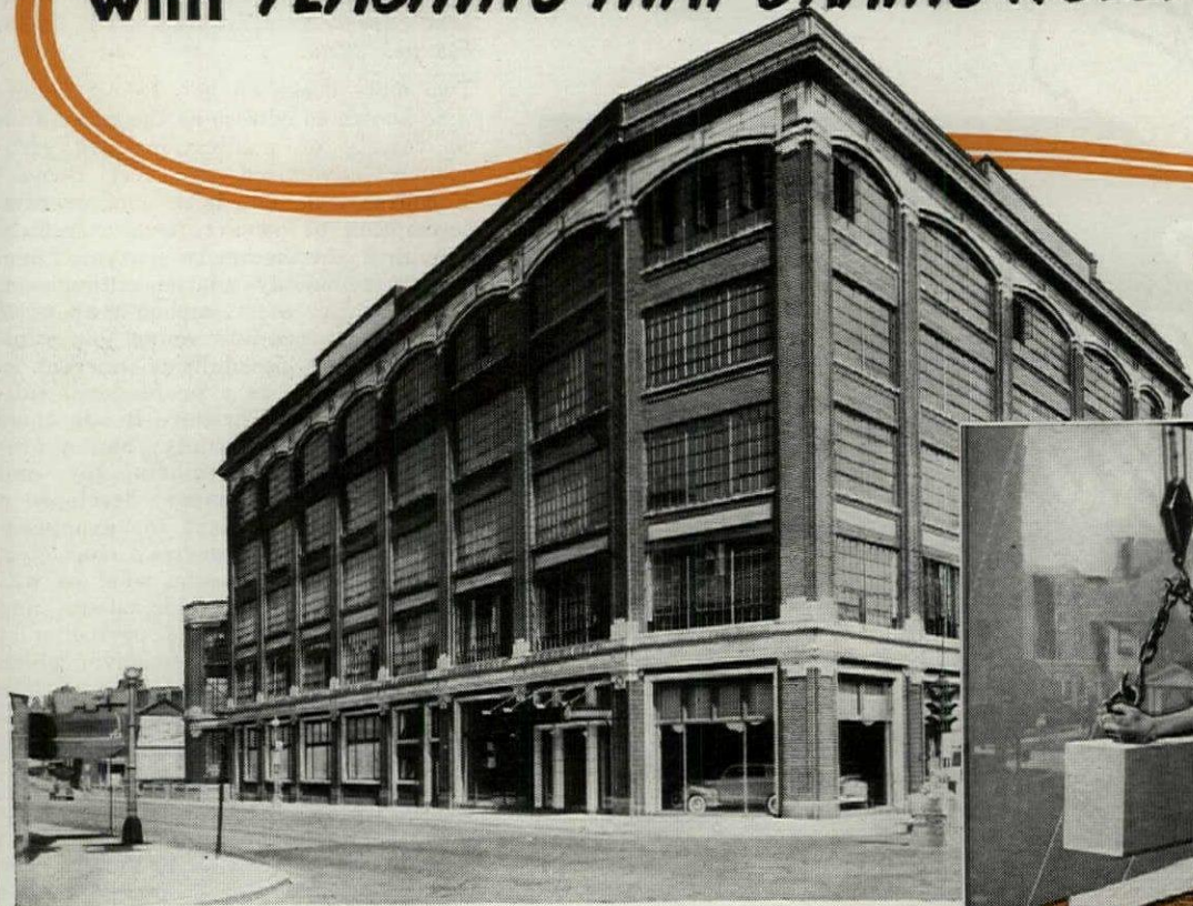
Automotive branch plant, in which 6,000 lb. of Anaconda Through-Wall Flashing were installed by Mandel Roofing Company, Pittsburgh, Pa.
