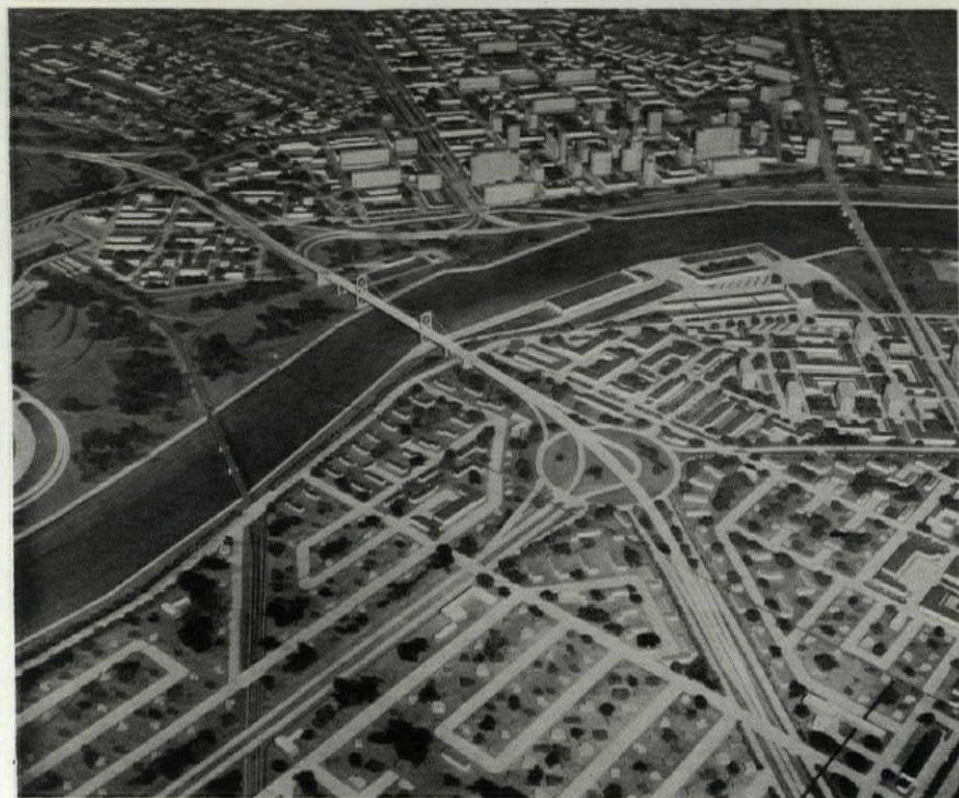
The aerial views (above) show Toledo, Ohio, and a model for replanning. The present crowded city is contrasted with the "congestion-proof" reconstruction proposed by Geddes. The photograph on the right shows his proposal for a more open downtown area—three-story flat-top office buildings predominating. Most of the taller buildings shown are existing structures.
