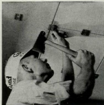
Of course, the Floating Wall System is also used for the ceilings.
