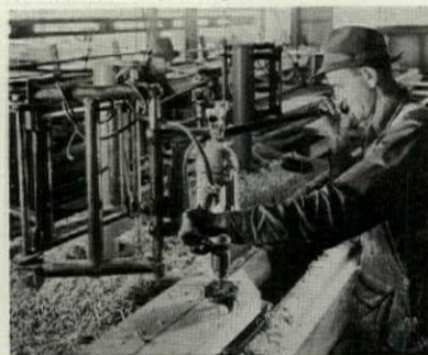
LEFT, fabricating timbers for split-ring connectors. RIGHT, long-span bowstring trusses of timber assembled with connectors; top and bottom chords are laminated, glued.
