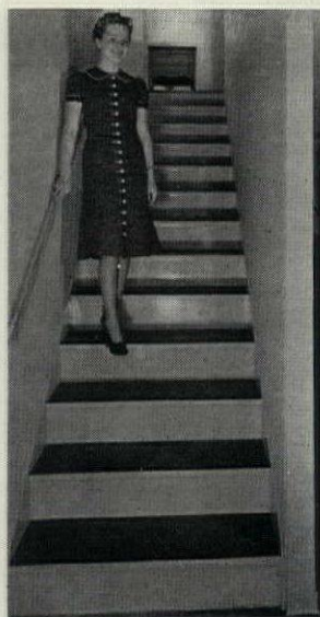
Steel stairs, prefabricated, installed as a single unit.
