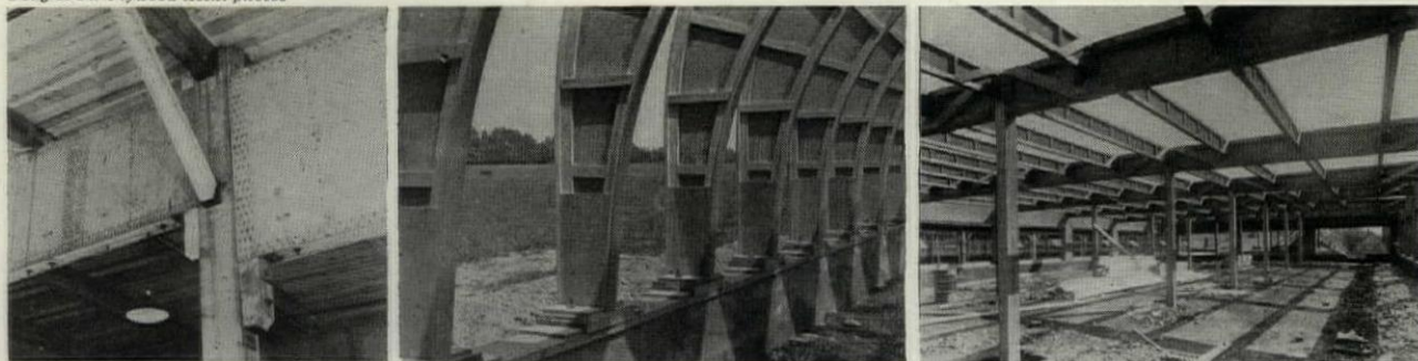
LEFT, composite wood girders in plant for R.C.A. Mfg. Co., Camden, N. J., with laminated flanges and nailed plywood webs. CENTER, composite construction of wood arches, with lumber flanges and plywood webs, nailed and glued. RIGHT, composite beams with lumber flanges and plywood webs.
