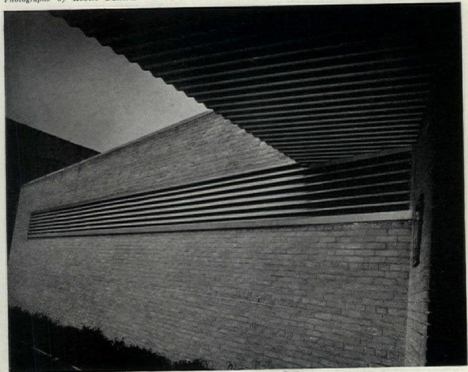
A CONTINUOUS LOUVER outside the dormitory is both a light baffle and a ventilating device.
