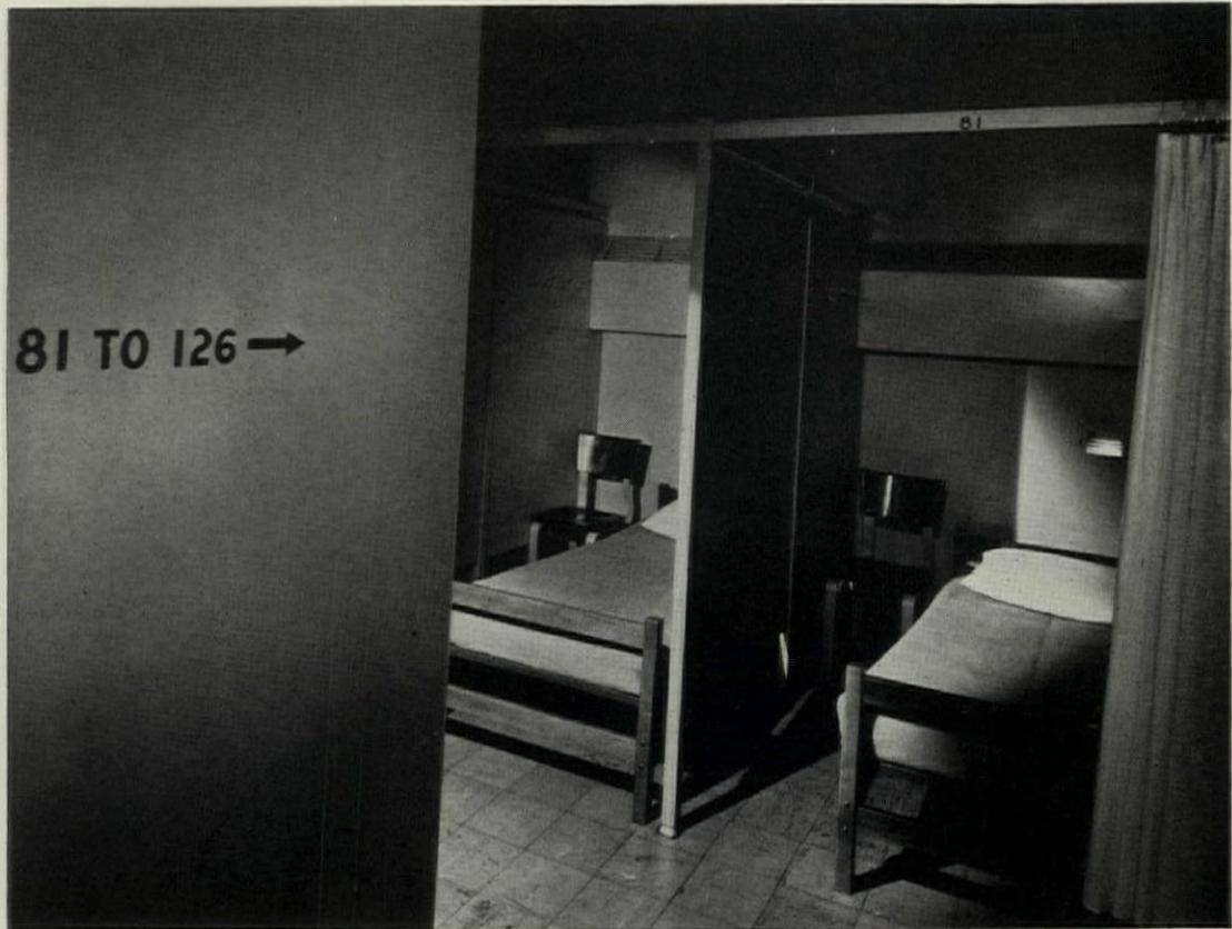
TYPICAL DORMITORY SPACE—metal partitions, asphalt tile floors, plaster walls and ceiling.
