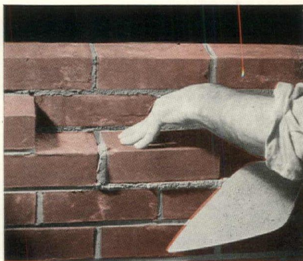
joint. The more plastic the mortar, the easier the work. Try this with Brixment mortar!
