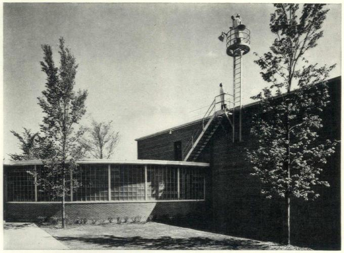
A curved wall of Insulux Glass Block transmits diffused daylight in abundance to the product development model shop in Benjamin Electric Mfg. Company's splendid new laboratory at Des Plaines, Illinois. The free-hand abstract pattern of 12" and 6" square
