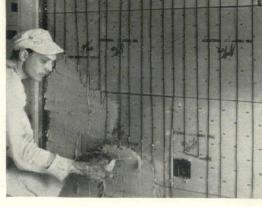
FIGS. 6, 7, 8, 9-Heating elements must be installed over non-metallic plaster base when
