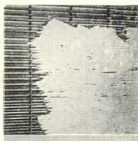
Above: The scratch coat is forced through Milcor Metal Lath so that it is keyed on both sides of the steel reinforcing.
