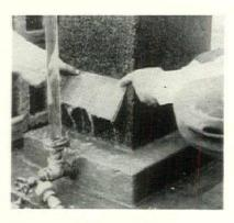
Hollow, highly porous cinder concrete block columns used in recent tests of Aquella waterproofing, built, and Aquella applied to one, with common labor. Treated column (white) held 8 ft of water (approx. 500 lb per sq ft——almost 50 times as severe as NBS' 10-lb test) while untreated column could not be filled above 18¾" because water seeped out at 2 gal per min.
