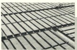
Here is a Ceco job illustrating precision formed joists. Note the constant width and accurate alignment from one end of the building to the other. Ceco workmen know how to eliminate concrete leakage and insure proper execution of the structural design.
