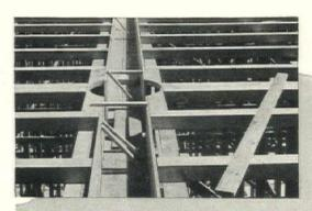
Simple open-wood centering makes Meyer Steelform construction economical and fast. The centering may be re-used from floor to floor. This eliminates extra lumber and saves time.
