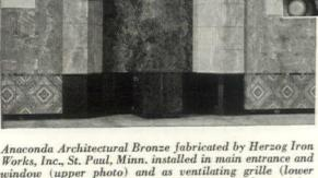
Works, Inc., St. Paul, Minn. installed in main entrance and window (upper photo) and as ventilating grille (lower photo). Entrance shown is one of three, each requiring about 8,000 lb. of Anaconda Extruded Shapes and special Ingots for castings of matching color.
