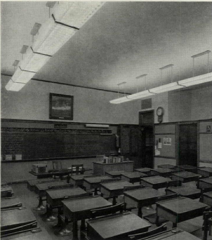
Fig. 5. School relighting programs require careful planning to achieve the objective of sufficient, comfortable, healthful light on desks and chalkboards, at minimum over-all cost. In the example illustrated, two rows of louvered, direct-indirect fluorescent luminaires provide over 40 foot-candles (average) on desks. Bottom louvers shield lamps at normal viewing angles and also prevent accumulation of dirt, bugs, and paper wads.
