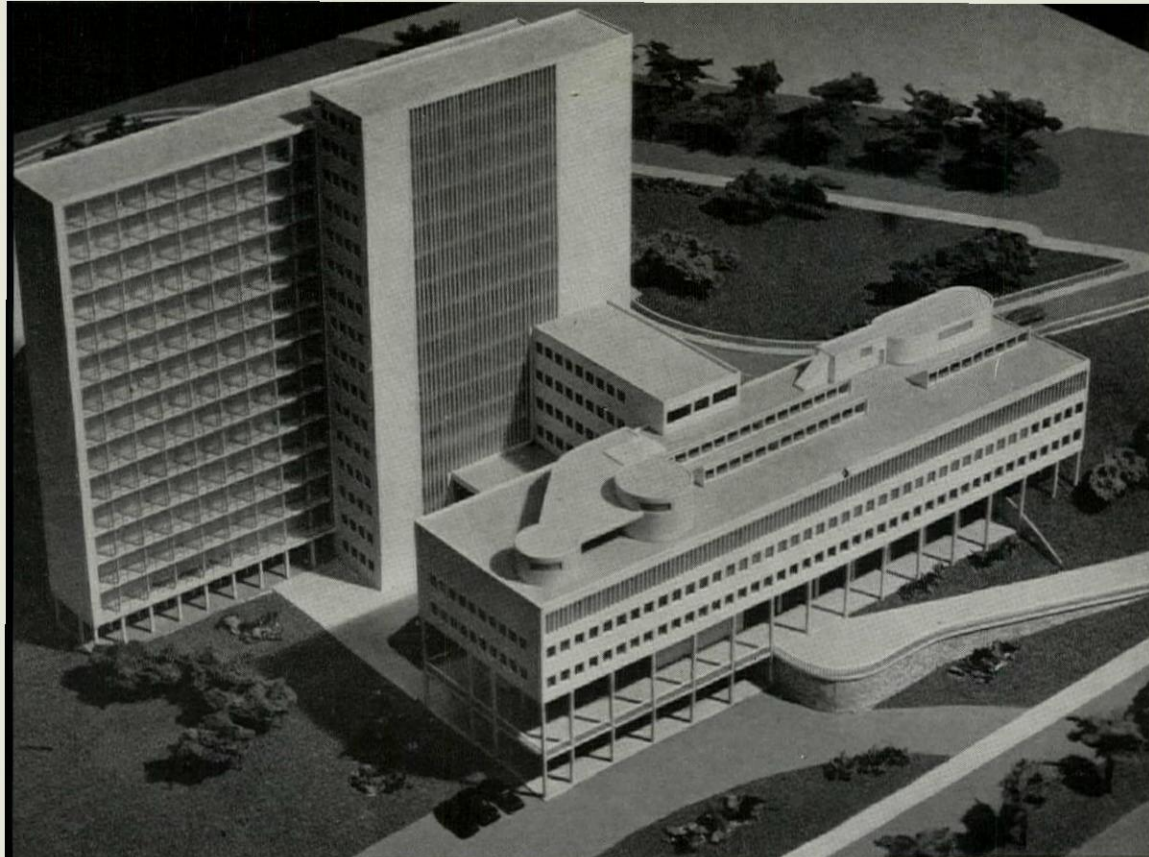
North (sunny) facade of the projected University Maternity Hospital for Sao Paulo, Brasil (Rino Levy, architect) is essentially a composition of various sun control devices. These include minimum openings, deep porches and balconies, and a grill-work of vertical louvers, utilized in accord with the needs of interior space for sun and light penetration.
