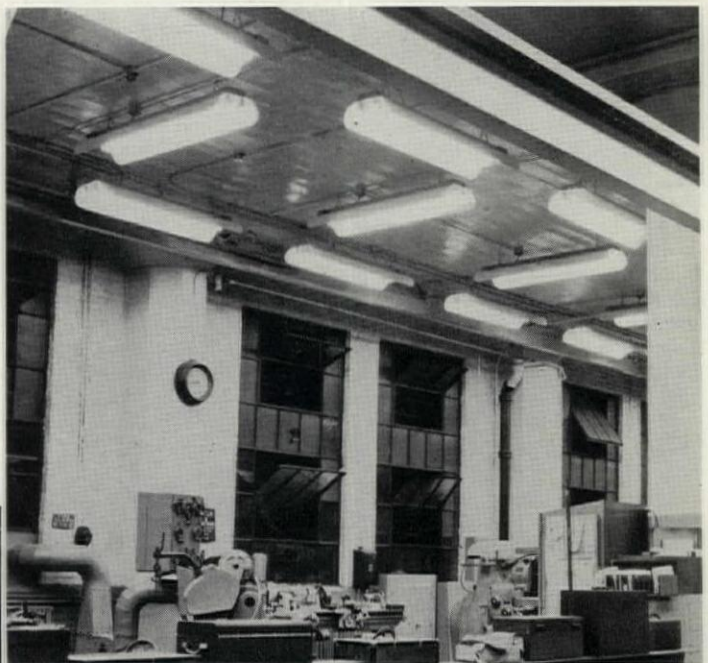
Fig. 10. In a tool room, machinists must frequently use micrometers, steel scales, and micrometer adjustments on machine tools. Each is a difficult seeing task; one of the functions of lighting is to improve visibility for such purposes. By installing luminaires in two directions in a grid pattern, the graduated markings and numbers are easily seen against a luminous background which is a reflection of the low-brightness, large-area fluorescent sources. In this case visibility depends upon reflected luminaire brightness rather than on foot-candles on the work.
