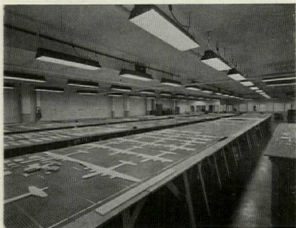
PLANT LAYOUT ROOM with unit fluorescent fixtures; note the blackout panels, inside the windows along the far wall.
