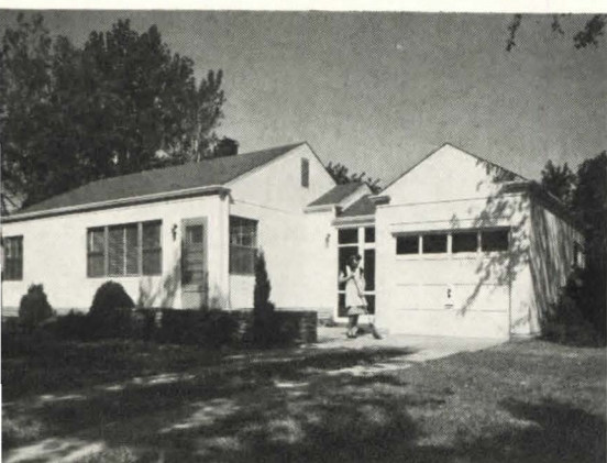
"Aluminum" house developed by the Butler Manufacturing Company, called "Boulevard Home," employs 2,300 lbs. of steel, principally in the roof framing, with wall panels of aluminum joined by a simple wedge. Interior may be any finish desired; rough floors are wood.
