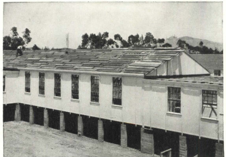
Cemesto walls on one of the sections of the large Naval Hospital at Corona, Calif.
