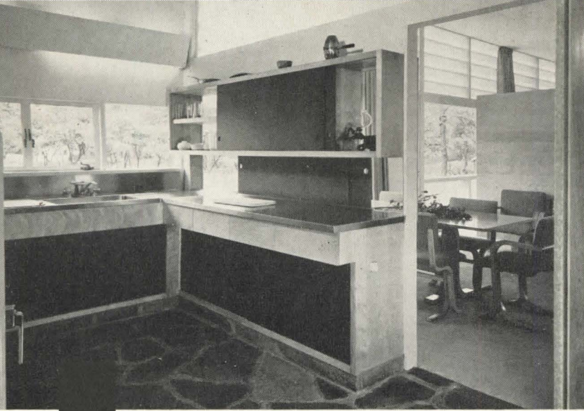
11 . . . Kitchen. Stone floor, plywood walls; sliding cupboard doors, hard fiberboard.
