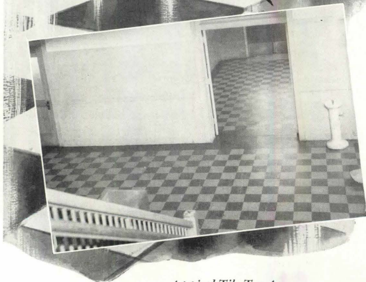
A typical Tile-Tex Asphalt Tile installation in a school corridor.
