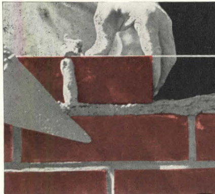
The brick should be shoved into place so mortar oozes out at the top of the joint.
