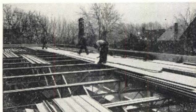
Application of "Ferrobord" Steeldeck
