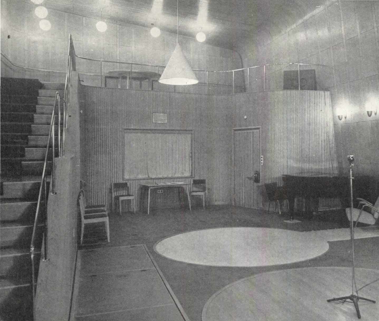
DRAMA. For underfoot noises: 4 types of floors; concrete, carpet, and wood stairs; crushed rock, etc., in bins under floor panels (left).
