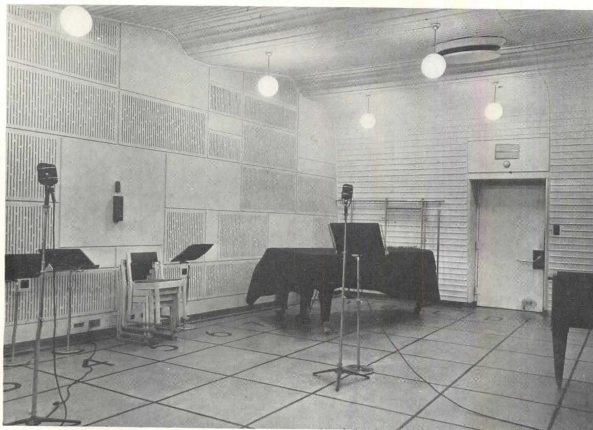
CHAMBER MUSIC STUDIO is similar in treatment to the small orchestra room; bent-section ceilings; walls of perforated acoustical panels.
