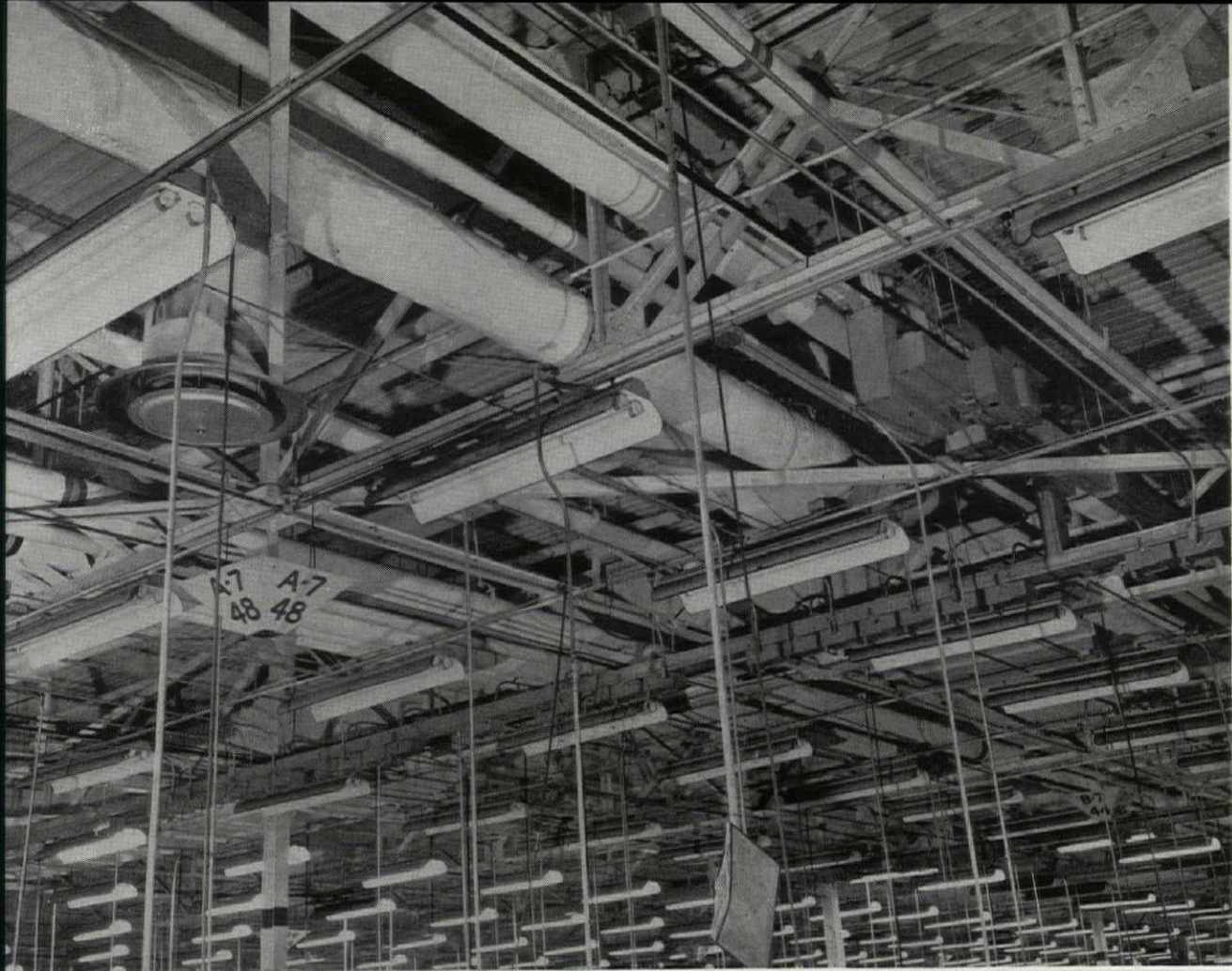
THROUGH FACTORY ROOF TRUSSES are distributed electric power, compressed air, high-pressure steam, other services.
