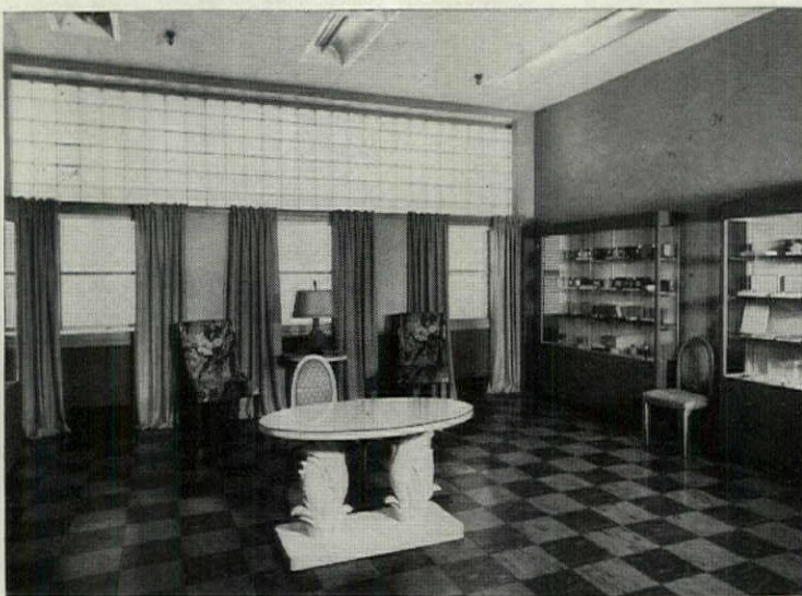
Insulux Prismatic Glass Block turns light to ceiling for re-direction into this second-floor display room. Drapes over windows can be entirely drawn without loss of daylight in room. Same type panels give fine working light in factory areas.
