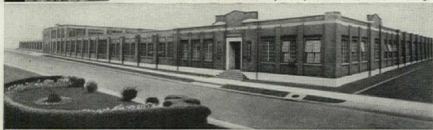
Main office and factory of Jamestown Metal Corp.
