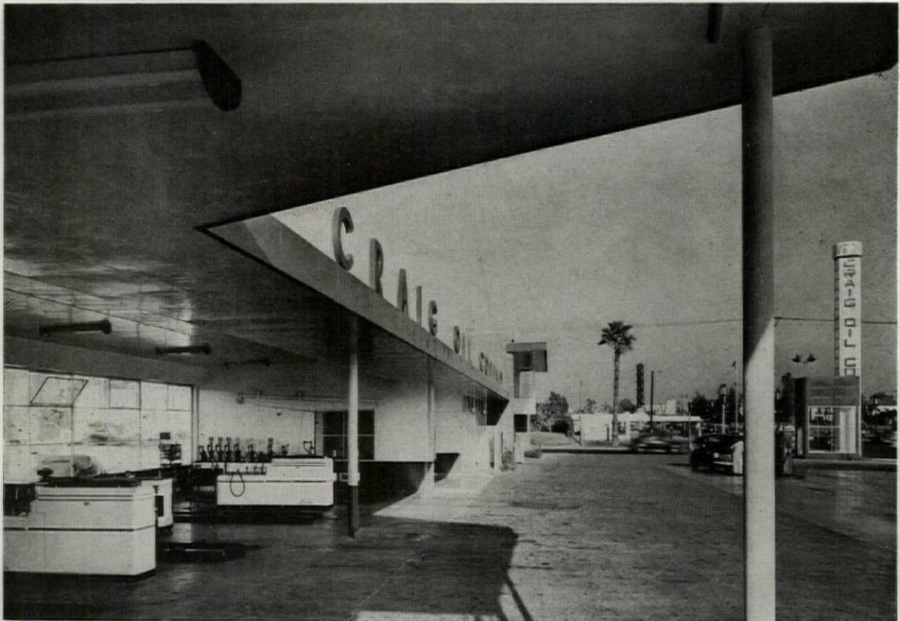
VIEW FROM ROOFED TERRACE LOUNGE for patrons, showing lubrication racks, fire wall, and at right in distance, sign pylon. Roof is suspended from exposed light steel trusses to obtain a clean, flat ceiling, and has mineral wool insulation. Construction is steel, surfaced with porcelain enameled steel sheets, red and white in color. Roofing is perforated asbestos.
