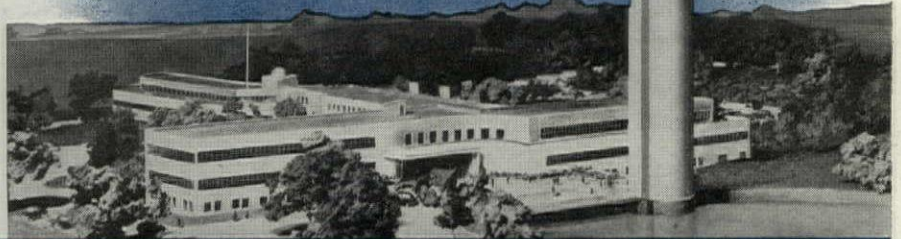
Federal Telecommunications Laboratories, Nutley, N. J. Largest all-metal commercial group in the world. Architects—Louis S. Weeks, N. Y. C. (groups 1 & 2); Giffels & Vallet, L. Rossetti, Detroit (groups 3 & 4).
