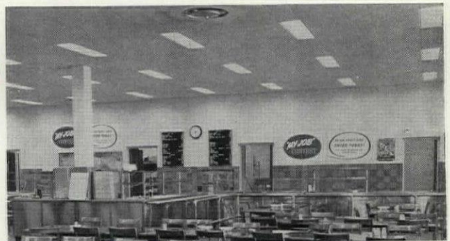
CAFETERIA (also office space) has recessed fluorescent fixtures.
