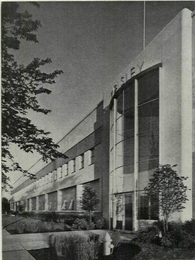
Ground to roof facade of Allen B. Wrisley Company, Chicago, has continuous panels of Insulux Prismatic Glass Block. Three face patterns and approximately 4500 glass blocks provide the ultimate in daylighting this modern and progressive plant. Architects: Fugard, Burt and Wilkinson, Chicago Ill.
