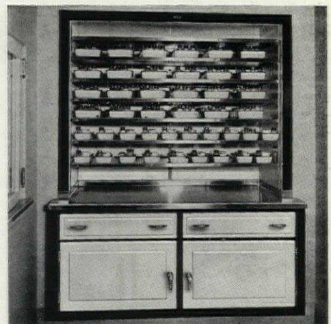
Recessed cabinet in maternity department. Upper section open and fitted with adjustable stainless steel shelves for holding mothers' treatment trays.
