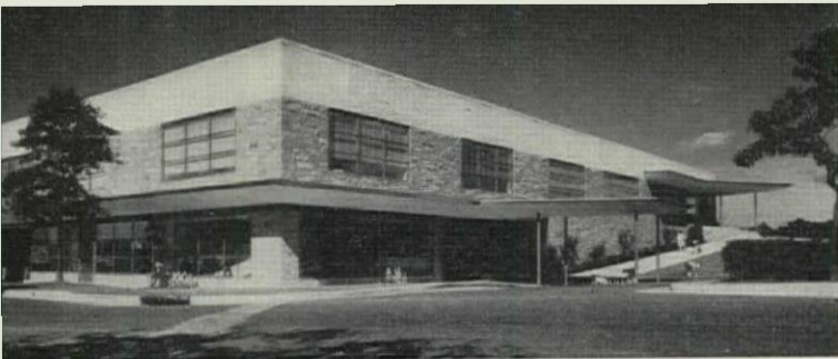
VIEW FROM SOUTHWEST: Cavity wall construction—exterior with granite; 2-in. air space; interior with terra-cotta block.
