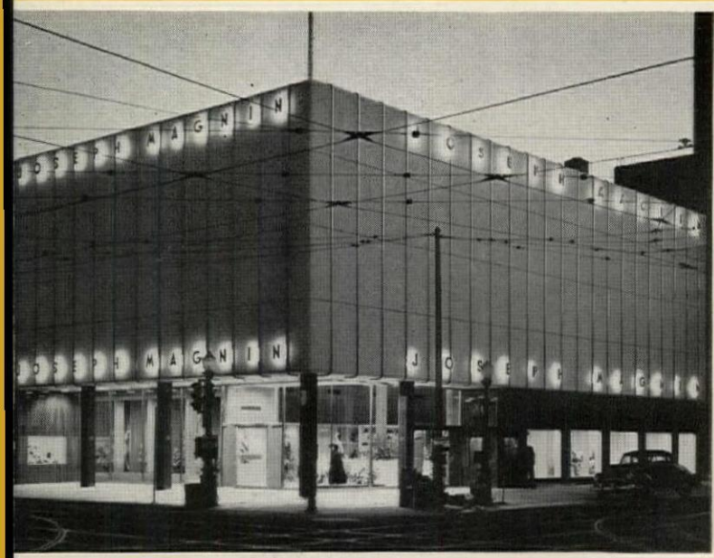
Joseph Magnin Co., Inc., Sacramento, Calif. Pozzolith Architectural Concrete. Archt.—Harry J. Devine, Sacramento, Calif. Structural Engineer—Ernest D. Francis, Sacramento, Calif. Gen. Contr.— Swinerton & Walberg Co., San Francisco, Calif.
