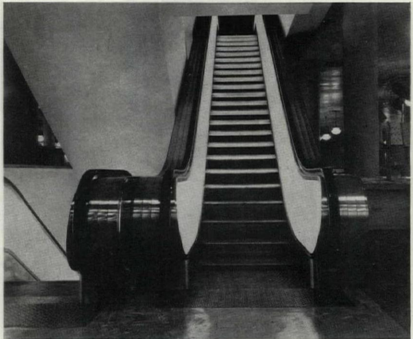
ANOTHER NEW DEVELOPMENT in this field is the illuminated balustrade applied by Otis to the Escalators recently installed in a Dayton, Ohio, department store. The entire interior paneling of the balustrade consists of frosted tempered glass, lighted from behind by cold cathode tubing. This installation was designed by Eleanor Le Maire as an improvement on the usual overhead lighting.
