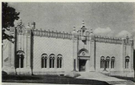
BEFORE: Original building, completed in 1927; Long & Thorshov, architects. For work this firm is NOW doing, see the special feature in our next month's issue.
