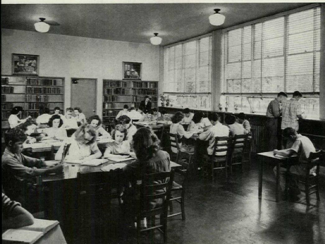
THE LIBRARY. Construction allows the big windows to reach practically to the ceiling line. Asphalt tile is the floor covering here, as it is throughout the building.
