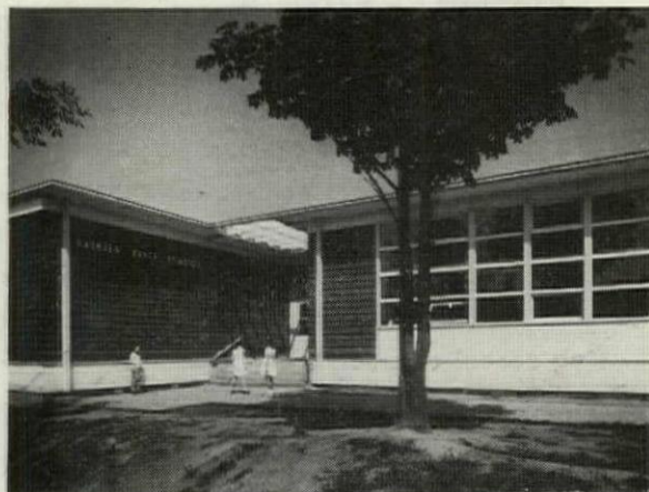
THE BUILDING is of frame construction, with red cedar outside and wallboard within.
