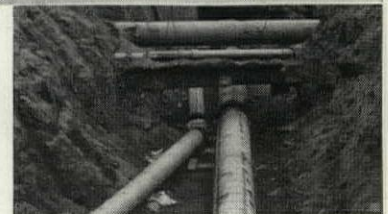
Ric-wiL Units being installed in shallow trench at Fresh Meadows
