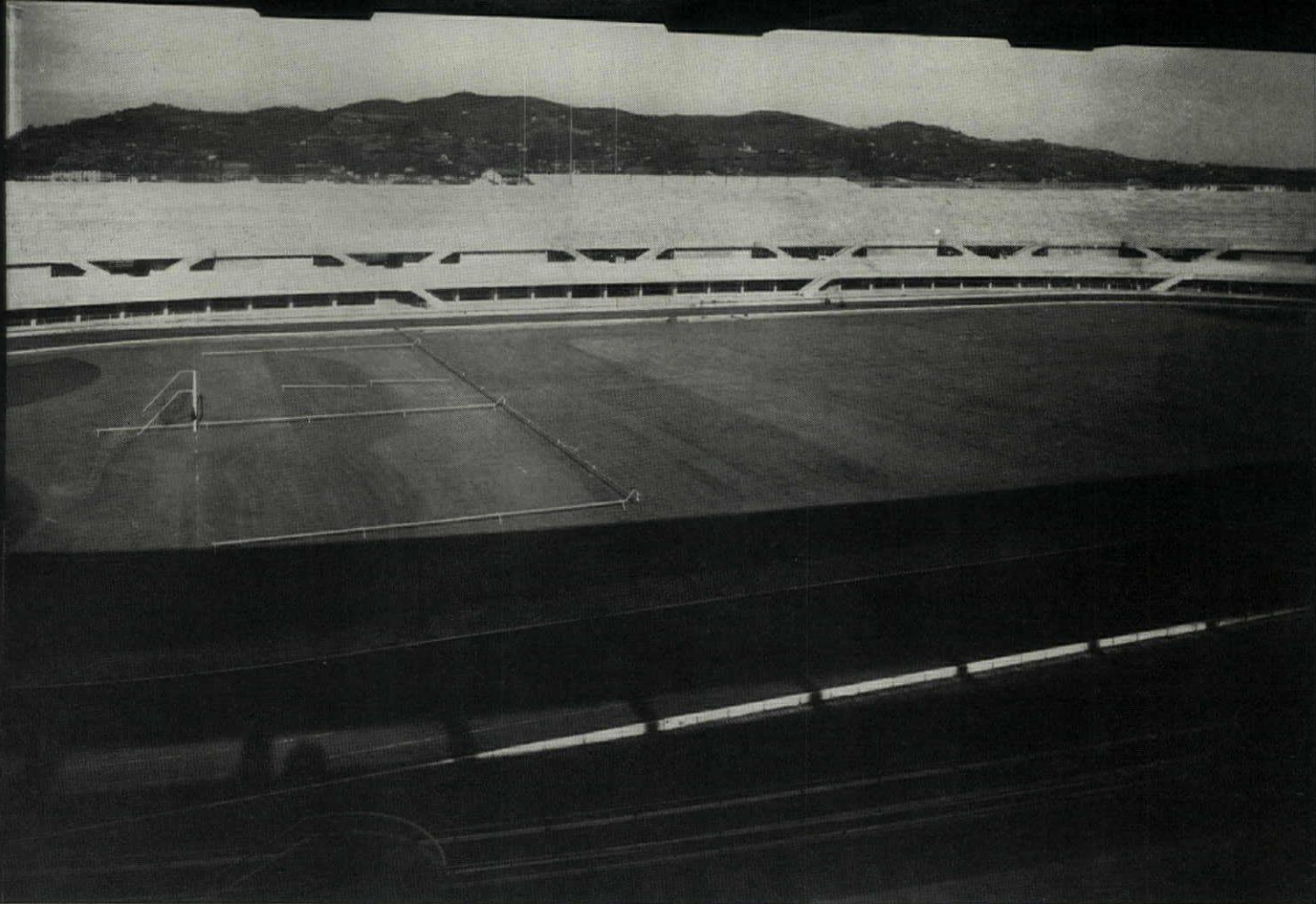
VIEW FROM UNDER THE CANTILEVERED CANOPY of the grandstand. In addition to a football field, the grounds include a six-track course for track events; two long-jumping units; four areas for high jumping and pole vaulting. The stadium seats 45,000 persons.
