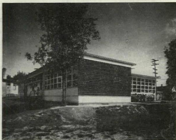
BLANKED END WALL of west kindergarten is because of distracting, near-by view.
