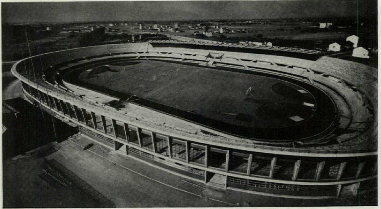
THE ELLIPTICAL BOWL completely surrounds the field. Twenty main entrances feed into a mid-level aisle on the field side and thus, via stairs, either up or down to the tiers of seats.
