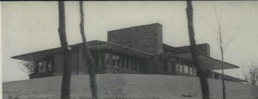
HOUSE of deep red brick and stained oak, by E. J. Mutrux & W. A. Bernoudy, architects, was the first in St. Louis (1940) to use hot water radiant heating. It is now the Louis E. Mutrux residence.
