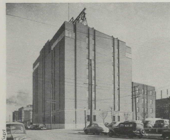
CENTRAL OFFICE BUILDING for Monsanto Chemical Company is a new "semi-windowless" steel and brick structure. To provide the same working conditions for all employees, it is uniformly lighted and air-conditioned throughout. The few windows provided by the architect, Walter J. Knight, are intended for emergency use only.
