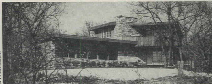
HOUSE of local limestone and stained oak, by Robert L. Fischer, designer, for himself and another faculty member at Washington University. Roofs can carry 1½" of water for insulation during hot summer months.
