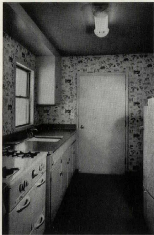
SHUTTER FRONT on kitchen counter drawers eliminates the usual drawer pull without complicating the work of craftsmen.
