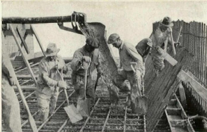
Pozzolith gave pumped concrete increased workability, easy placeability, good cohesiveness. Milwaukee Sewage Disposal Plant.
