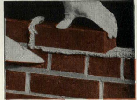
So that the mortar oozes out at the top of the head joint.
