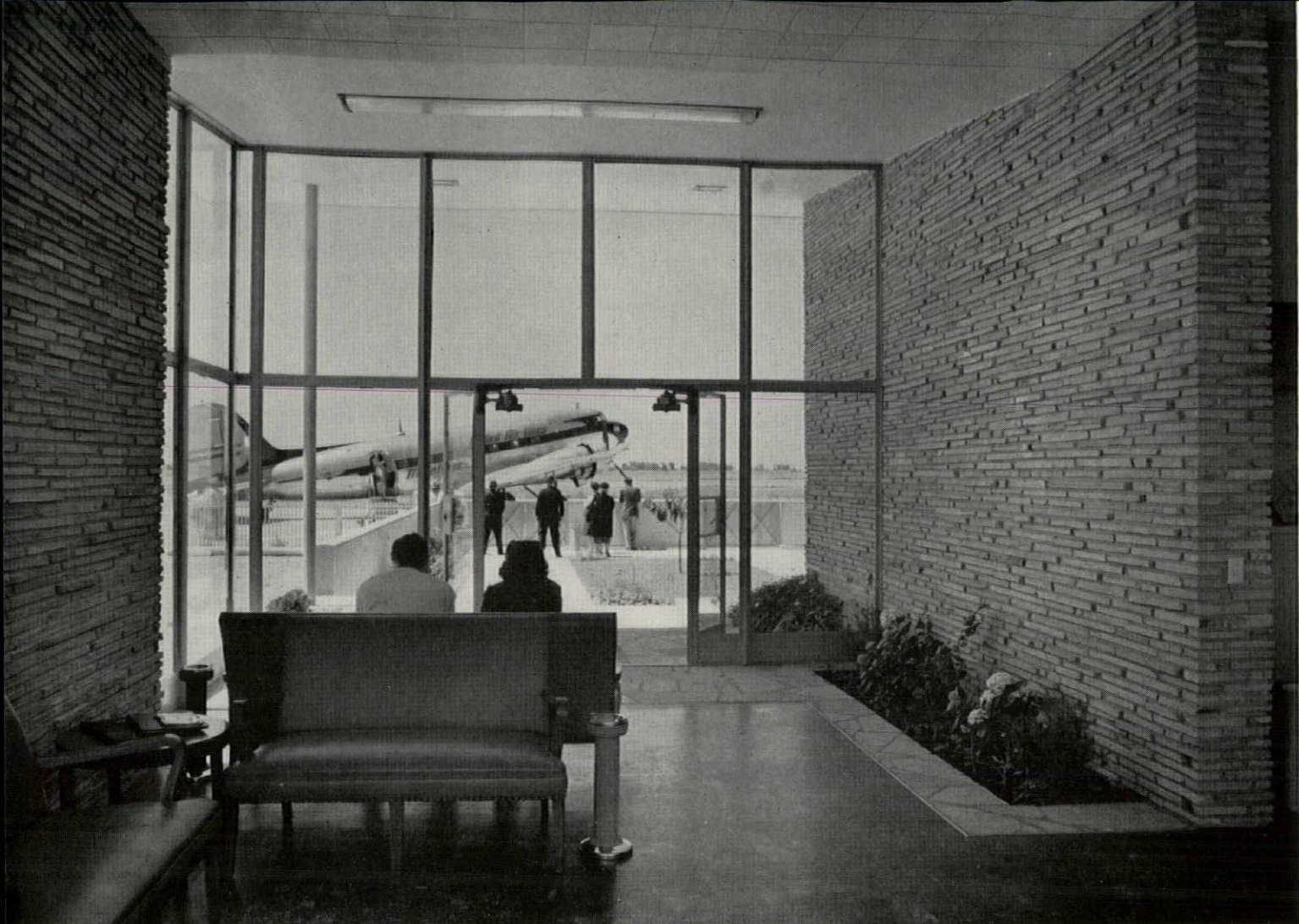
View from waiting room out to field. Copper radiant heating coils are embedded in the asphalt-tile-surfaced, concrete slab floor.
