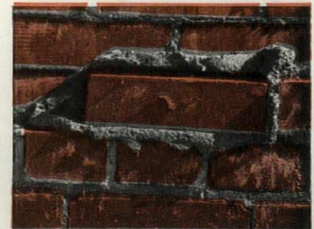
So that the mortar oozes out at the top of the joint.
