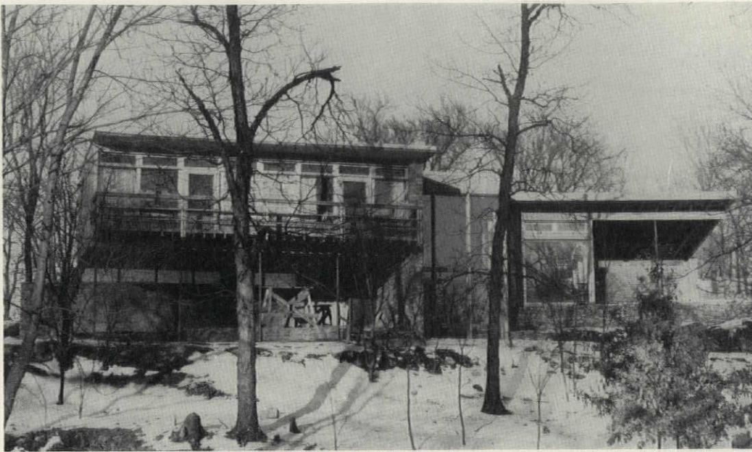
Local stone masonry; "fairly standard framing" on a 4-ft. module.
