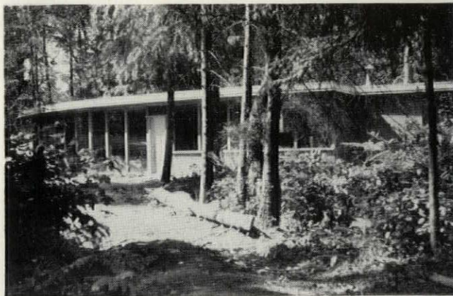
MERCER ISLAND, WASHINGTON: House. Bassetti & Morse, Architects. Wood-frame on concrete slab; integral radiant heat system. P/A will publish.
