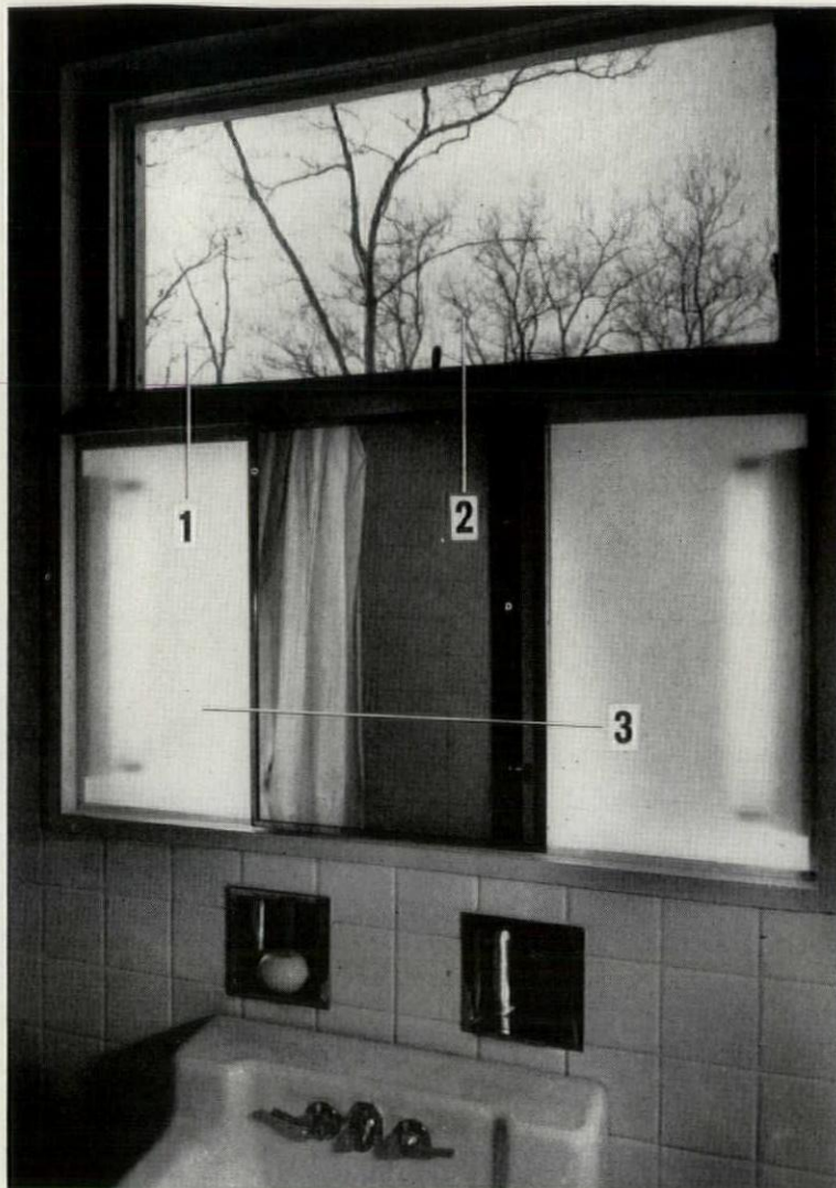
Medicine cabinet and fluorescent lights are built into a preassembled window unit. This makes possible more efficient utilization of bathroom space, provides good face-lighting by day or night, and since the architects have used the same detail in several houses a number of the units could be made up at the same time.
