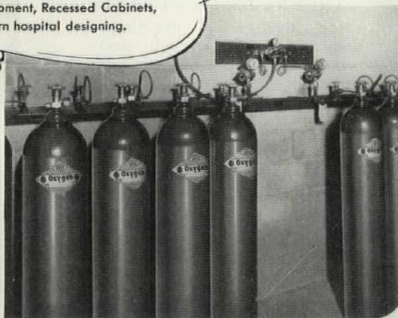
CENTRAL OXYGEN PIPING SYSTEM
