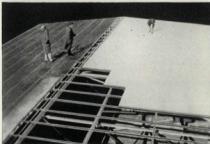
KAYLO ROOF TILE is simple to install, lightweight, saves steel.
