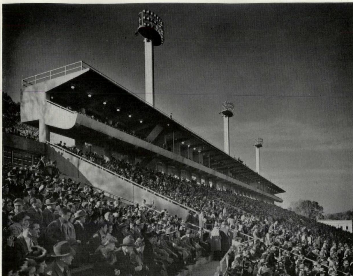
The new grandstands were built out from and above existing bleachers, increasing seating by 10,000.
