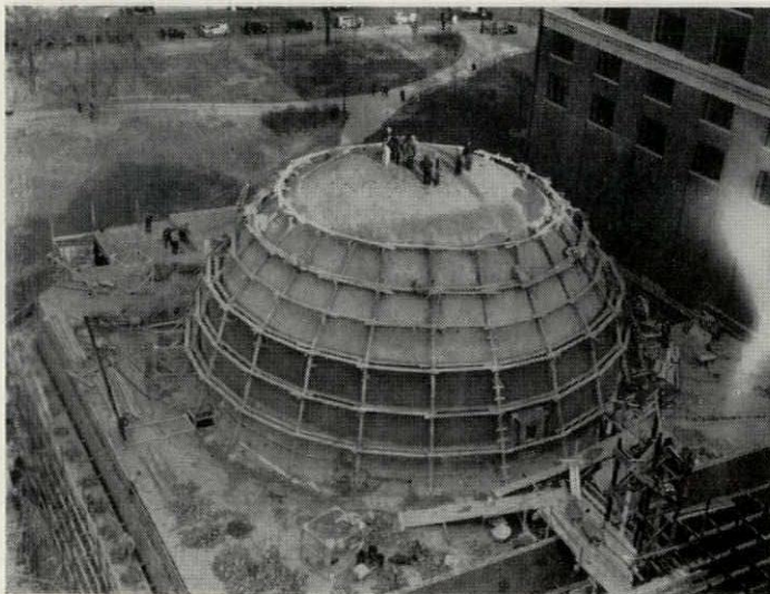
Hayden Planetarium, New York, has a spherical dome of gun-applied concrete over wood frame; construction occurred in early winter season.
