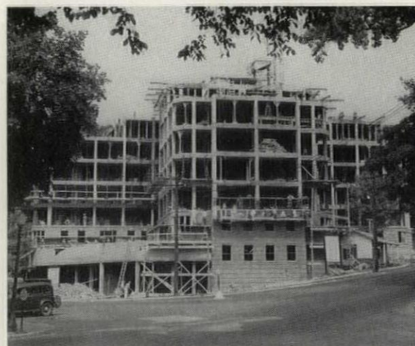
Popham Hall, Scarsdale, N. Y., apartment building, had to be rushed for early occupancy. Use of “high-early” permitted construction scheduling which saved both time and money—$1.45 per cu yd of concrete.
