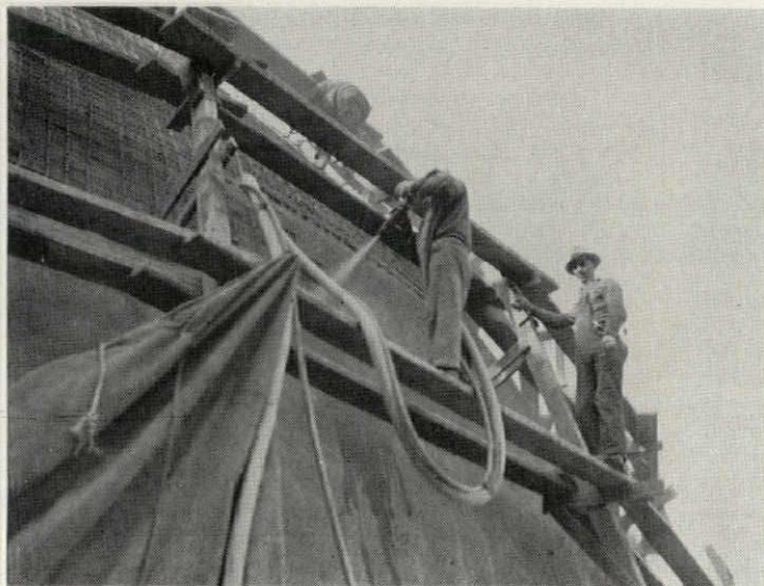
Hayden Planetarium, New York, has a spherical dome of gun-applied concrete over wood frame; construction occurred in early winter season.
