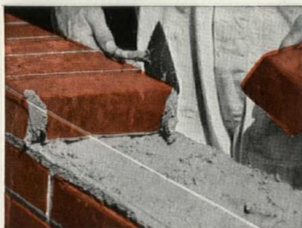
When mortar is spotted on both corners of the header brick,
