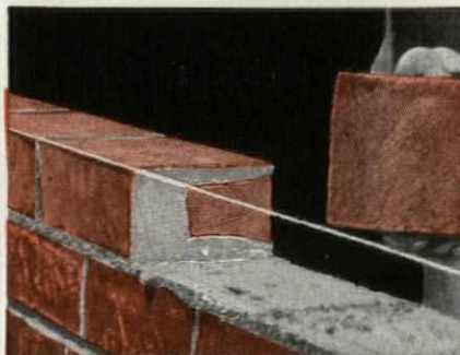
When mortar is spotted on only one corner of the brick, slushing seldom fills the voids.
