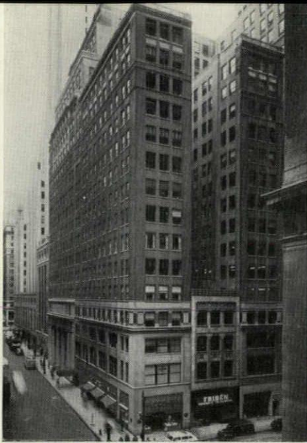
Building in New York City has facade of left wing coated with Corrosite; right wing is not. Prior to Corrositing, say owners, moisture penetrated wall and damaged interior plaster. Since Corrositing (two coats, June 1947) there has been no moisture penetration, no discoloration of brickwork.
