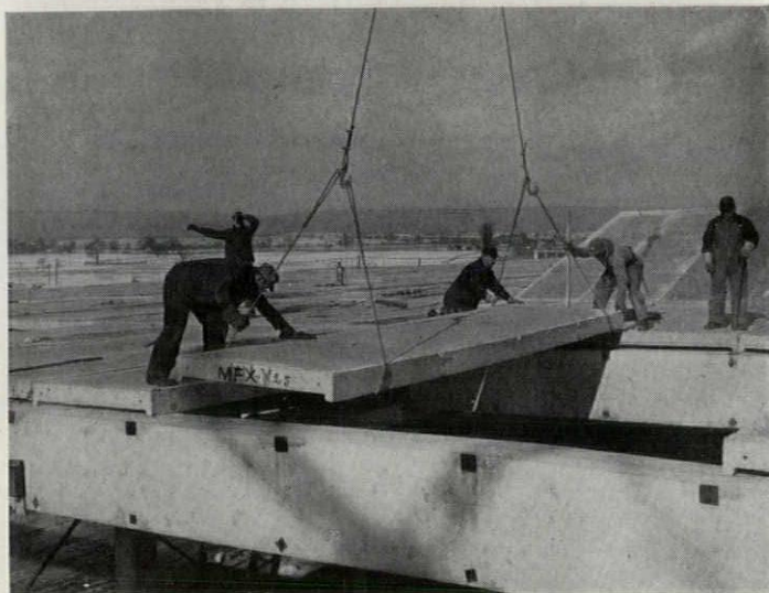
Prefabrication in concrete has also benefited from use of high-early strength Portland cement. Photos show (upper left) foreground, roof panels poured in forms on the ground at the site, and, background, being loaded on a truck. Upper right, placing prefabricated framing; forms were clamped around joints and joints poured. Lower left, frame nearly assembled, roof panels stacked ready for installation. Note that the season is winter. Lower right, placing roof slabs. (Naval Supply Depot, Mechanicsburg, Pa.)
