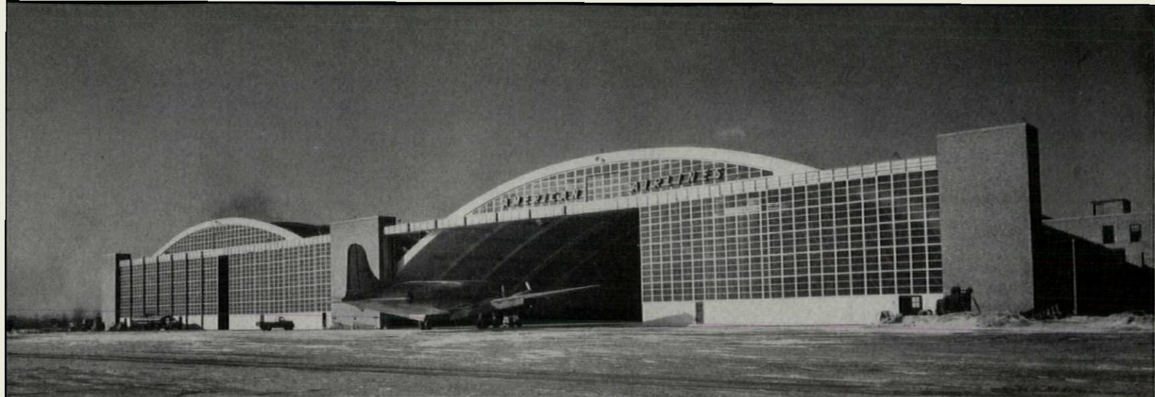
Thin-shell concrete hangars for American Airlines, Chicago, have the tremendous clear span of 257 ft between vertical walls. In construction . . . . .
