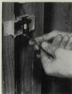
Installing: left, mounting 25v transformer; center, installing switchplate in lightweight wall box; right, installing low-voltage wiring. Note: no armor or conduit.
