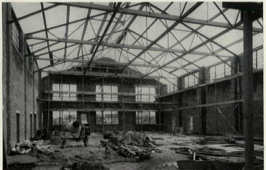
In this new building for F. W. Berk & Co. in Wood Ridge, N. J., manufacturers of chemicals, the owners expect a more accelerated corrosion problem than is normally encountered. Corrosite is being applied to all structural steel and window sash in two coats. All machinery, piping, etc., will also be Corrosited.
