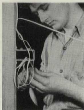
Installing: left, mounting 25v transformer; center, installing switchplate in lightweight wall box; right, installing low-voltage wiring. Note: no armor or conduit.
