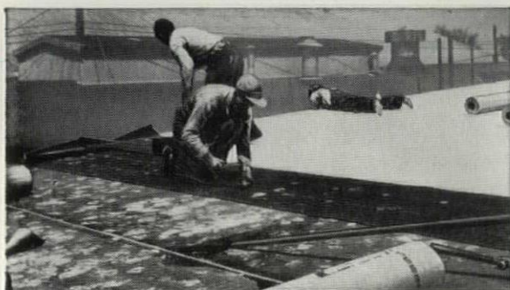
WHEN LAID , Kaylo Insulating Roof Tile is covered with conventional built-up tar or asphalt roofing. No other insulation is necessary.
