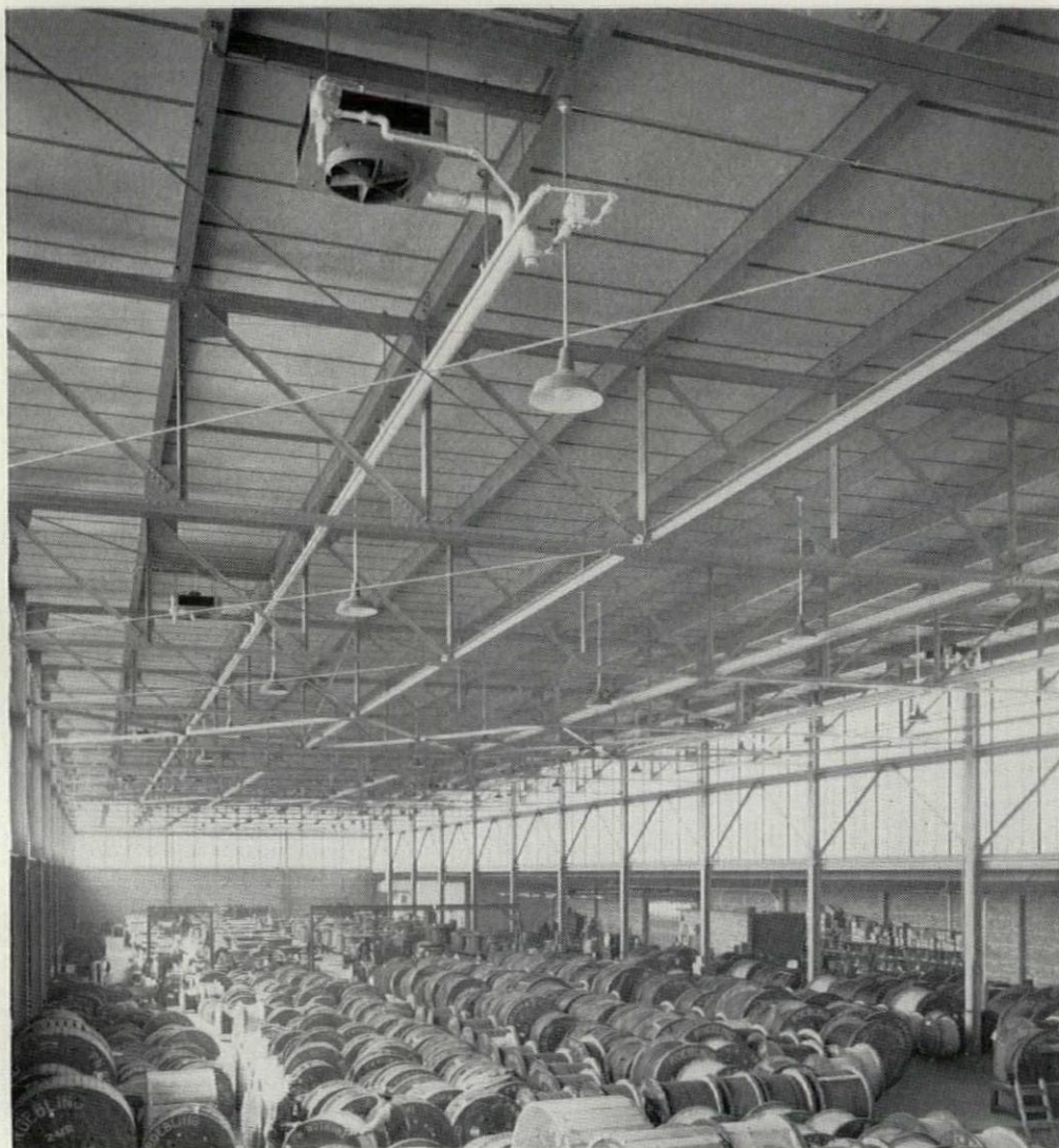
A CRANEWAY has subsequently been installed along this 72-foot-wide, 29-foot high bay.
