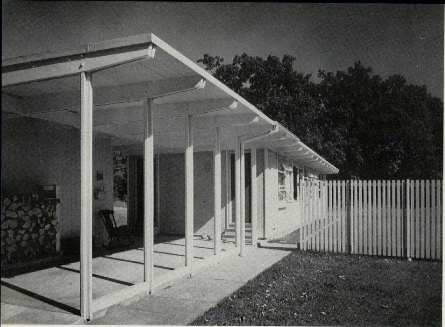
THE HOUSE is the structural scheme and vice versa. Shapes and spans were dictated by the system's economical limits.
