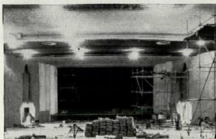
Truscon Metal Lath suspended ceiling partially covered with sprayed asbestos.
