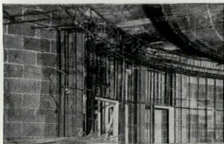
Construction details of Truscon Metal Lath ceiling and Cold Rolled Channel furring.
