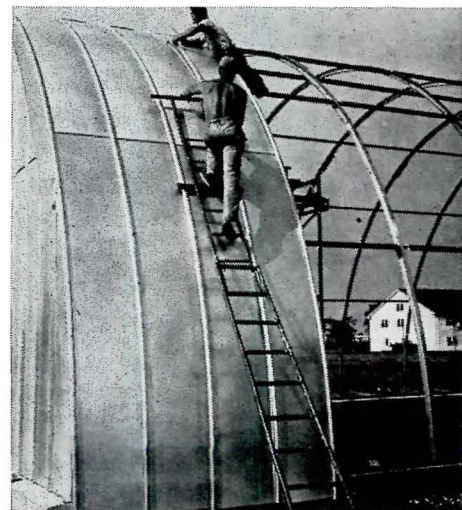
Left, Apostolic Church, Louisville, Ky., being constructed by members of its congregation. Studding, trusses reflective foil insulation, and siding are aluminum. Center, erecting structural aluminum framing (pre fab) for demountable midget auto race track designed by Leon & Lionel Levy, architects. Right, aluminum framing and sheet in a structure similar to the more familiar Quonset hut.
