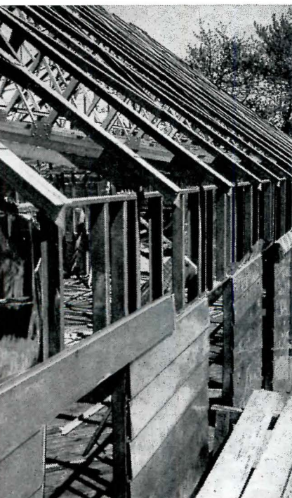
Left, Apostolic Church, Louisville, Ky., being constructed by members of its congregation. Studding, trusses reflective foil insulation, and siding are aluminum. Center, erecting structural aluminum framing (pre fab) for demountable midget auto race track designed by Leon & Lionel Levy, architects. Right, aluminum framing and sheet in a structure similar to the more familiar Quonset hut.
