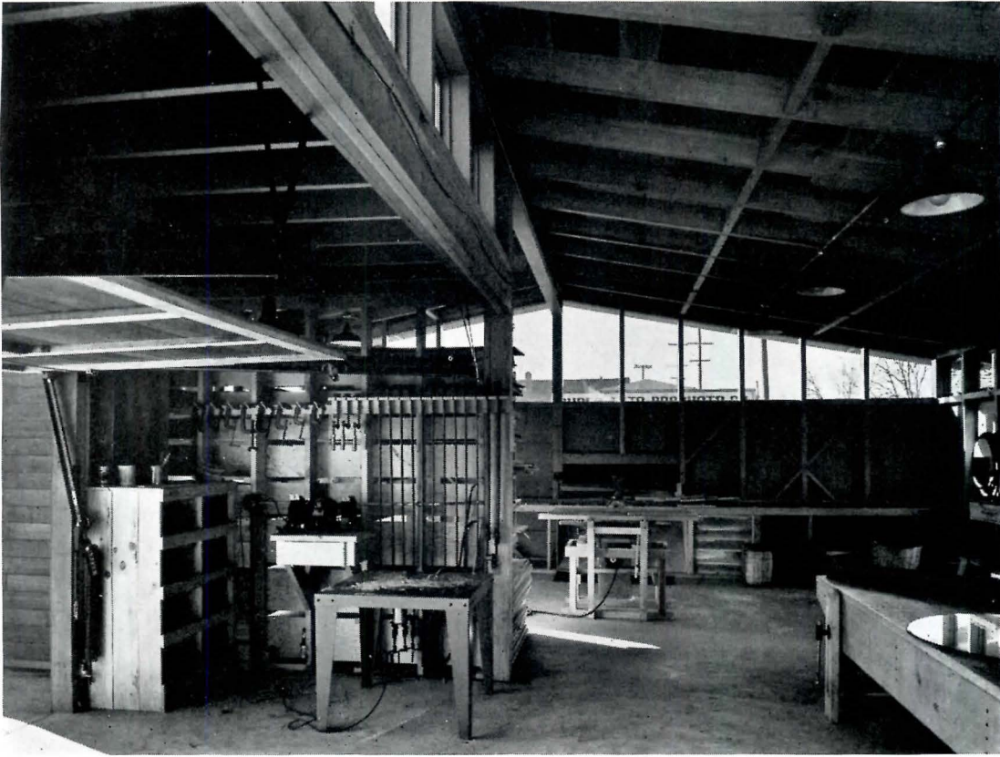
SHOP. Door at left opens to yard; stud walls spaced 32" on centers.
