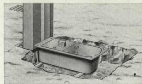
Floor closer ready for grouting in. On-the-job labor, special thresholds and other extras tend to make floor installation costly.
