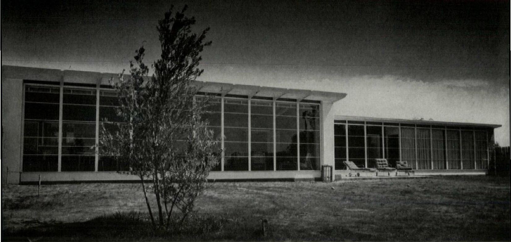
SOUTH WALL of windows transmitting sun and heat to the interior radiator wall. Overhang screens summer sun.
