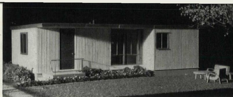
RELiance HOUSE, a prefabricated house with steel framing, has corrugated aluminum exterior surface, bonded on the interior to \frac{1}{2} " rigid insulating board; the curtain wall thus formed is a sort of semi-sandwich which helps resist wind loads. William Lescaze, architect; Paul Weidlinger, consulting engineer.
