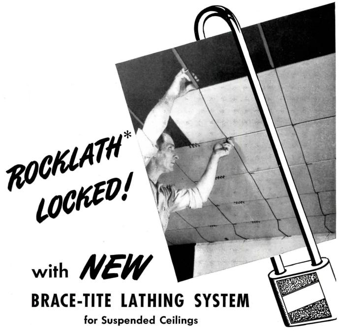
USG's new Brace-Tite Lathing System gives you all the advantages of Rocklath plaster base—plus the desirable features of suspended ceiling construction. It is easily adjusted to the contractor's working methods because no special tools are used, and no time-consuming training is required for either lathers or plasterers.
