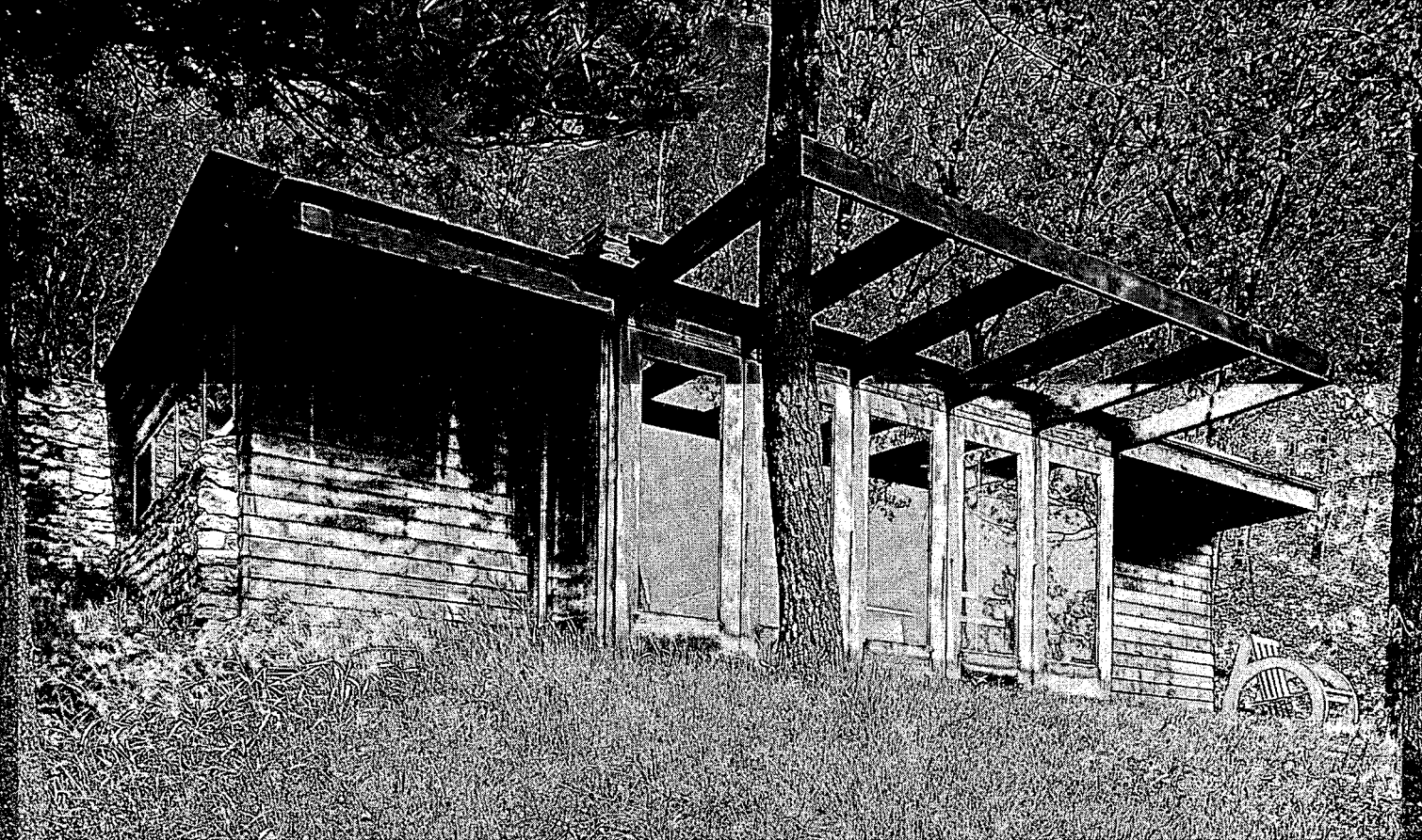
THE STONE RETAINING WALL returns around the north end, the slope of the ground allowing high windows above the work counter.
