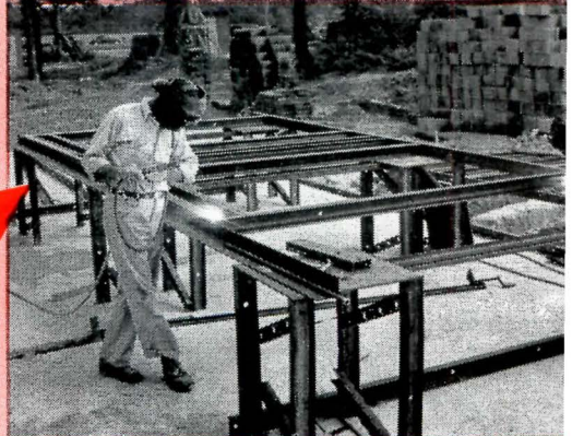
Accurately-sized Stran-Steel studs are now assembled into wall sections.
