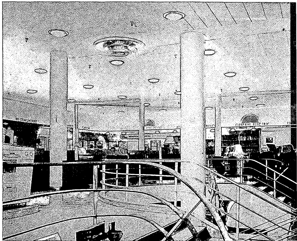
Air distribution outlets in The Hub, Baltimore, Md.; Tyler, Ketchum & Myers, architects; Egli & Gompf, engineers for the air-conditioning system.
