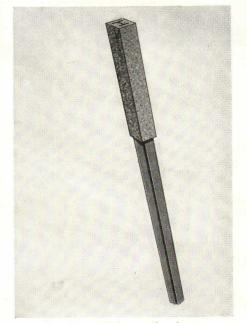
Corrosion of H-beam piles due to ground-water has been a major headache. Western Foundation Co. of Chicago has encased the upper 10 to 30 ft of steel piles in protective concrete. Above, protected 12"-53 Ib H-beam pile; below, driving piles for General Electric Turbine Plant, Schenectady, N. Y.
