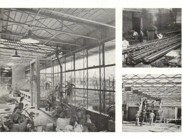
Wall framing was shopwelded in 30- to 40-ftlong panels; so were roof joists. In field, wall sections were clamped together and buttwelded, joists welded to them, creating a series of rigid frames. Shop fabrication, 90% of steel work, took three weeks, field erection, two weeks more.
