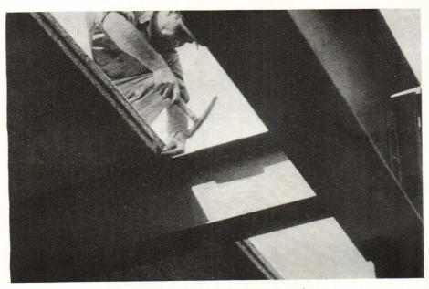
Roof slabs of Durisol (chemically stabilized wood waste bonded with Portland cement); one of several forms of this versatile material, the roof slab affords structural strength, lightness, dry construction, heat insulation, sound absorption, nailability. New to this country, Durisol has been satisfactorily used in Europe for 10 years. Durisol, Inc., 420 Lexington Ave., New York, N. Y.
