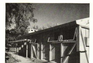
A multipurpose material fully exploited: exterior walls consist of a single sheet, 1-9/16" thick, of cement-surfaced fiberboard on an exposed frame; insulation is integral with construction.
