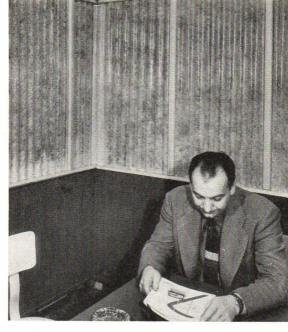
Glass fibers and plastics combined in a sheet material, rigid in one direction, reasonably flexible in the other. Prest-Glass, manufactured by Prest-Glass Corp., 8 E. 12th St., New York, N. Y.
