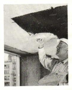
Plaster containing a new lightweight aggregate, Dantore, possesses insulating and fire-resistive qualities as well, does not interfere with plasticity or change plastering methods.
