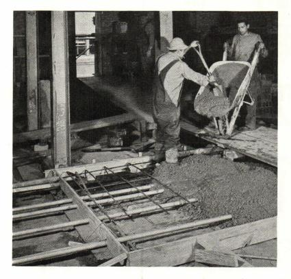
ELECTRUNITE E.M.T. is ideally suited for installation in concrete because it requires less space than ordinary threaded-type conduit. It is fully approved by the National Electrical Code for this and many other types of installation.
