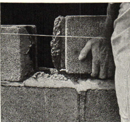
Method 2. A full head joint should be thrown onto one edge of the block already in place and also onto the opposite edge of the block to be placed.
