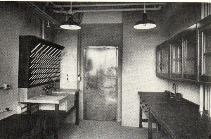
Physiology Laboratory: half-bay width. Ceiling-supported supply lines, each marked with individual identifying color, feed down behind wall-hung cases for attachment at bench height.
