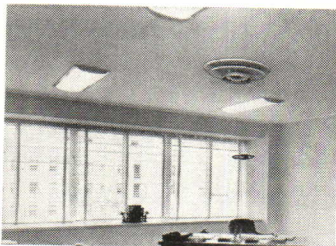
VENTURI-FLO CEILING OUTLET IN OFFICE
