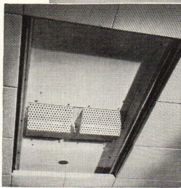
Concealed Multi-Vent Panel exposed by removal of six squares of metal acoustical ceiling.
