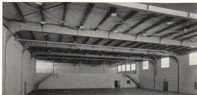
Another view of the Truscon Ferrobord Steeldeck in the Field House, Boy's Town, Nebraska.
