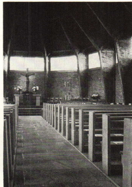
Prefabricated structural members and rubble walls, as used by Dr. Bartning for the Mannheim-Waldhof church (above) and for the Pforzheim church (below). The latter is model for 45 churches to be rebuilt with aid of Lutherans abroad.
