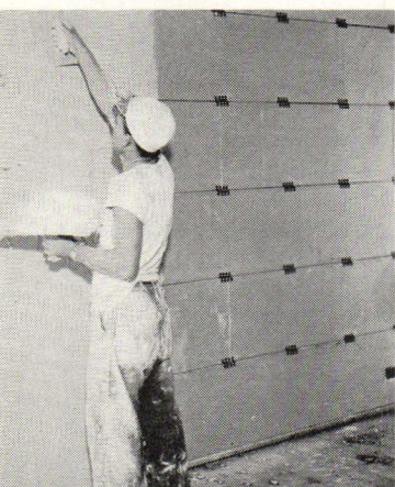
Typical brown coat application of Permalite - gypsum plaster. Compared with sand plaster, hawk load weight is reduced about two-thirds.
