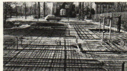
Radiant Panels installed in floor
