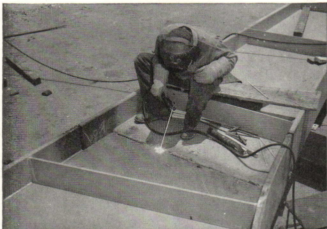
Fig. 1. Field welding truss sections to fabricate 200-foot span rigid frame, using 200-amp. Lincoln "Shield-Arc" Engine Driven Welders. Sections are lined up with a transit and tack welded prior to finish welding.
