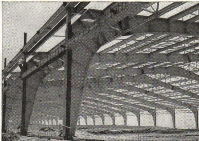
Fig. 2. All welded rigid frame Harbor Shed at Long Beach, California. Designed by R. D. Sandham under direction of R. R. Shoemaker, Chief Engineer, and R. J. Amar, Port Manager. Steel fabricated and erected by Pacific Iron and Steel Company of Los Angeles.
