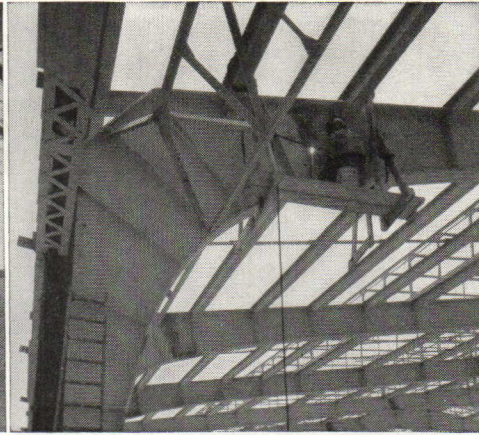
Fig. 5. Welding truss to hip girder. Butt joints are completed with ten passes on flange plate and two passes on web plate.
