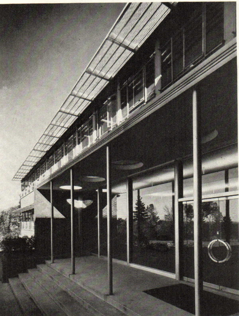
Entrance to west-facing main lobby and exhibit room is sheltered by the canopy shown in the photograph above. Above the window bands that light the offices is a continuous louvered, aluminum sunshade. Angle of the fins is set for total exclusion of sun on June 21.
