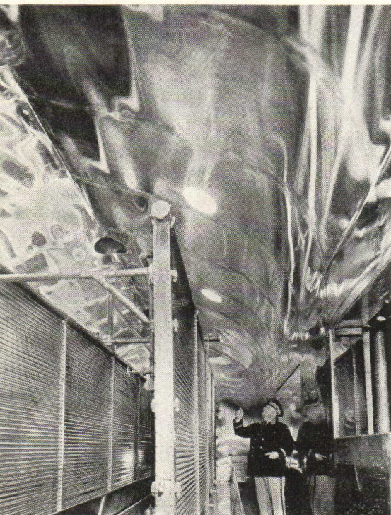
Above: downspout assembly showing details of stainless steel straps. Left: stainless steel walls in a beer cooling room of the Schlitz brewery, Milwaukee, Wisconsin.
