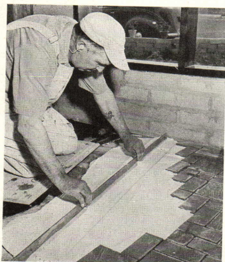
Left: workman spreads Expanset float-bed.
