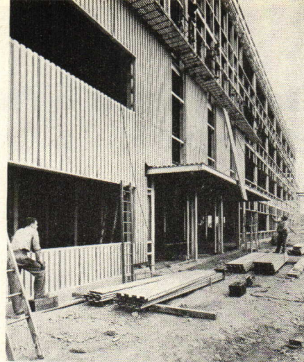
Left: installation of a stainless steel mullion in the Universal International Building, New York City.
