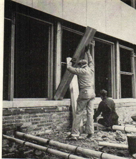
Left: installation of a stainless steel mullion in the Universal International Building, New York City.
