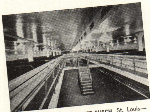
Starting tanks— ANHEUSER-BUSCH , St. Louis—fore-runner of many other concrete tanks at this great brewery.
