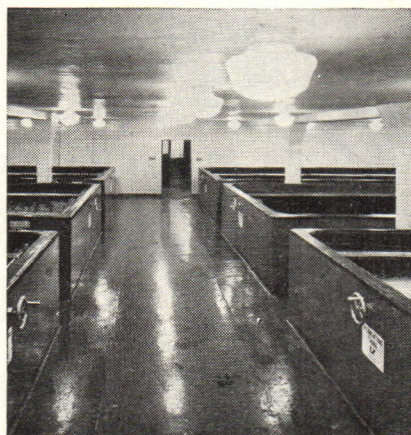
GRIESEDIECK BROS. Brewery, St. Louis—multiple-story closed fermenting tanks. Tanks, walkways, walls, stairways form completely monolithic structure.
