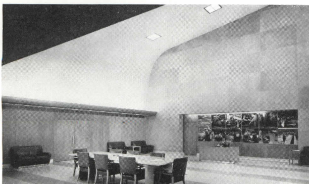
Lobby of office building is one and a half stories high, with curved acoustical ceiling. Walls—limestone and bleached mahogany; floor—terrazzo; door frames and trim—aluminum.
