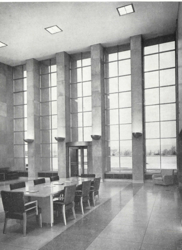
Lobby of office building is one and a half stories high, with curved acoustical ceiling. Walls—limestone and bleached mahogany; floor—terrazzo; door frames and trim—aluminum.
