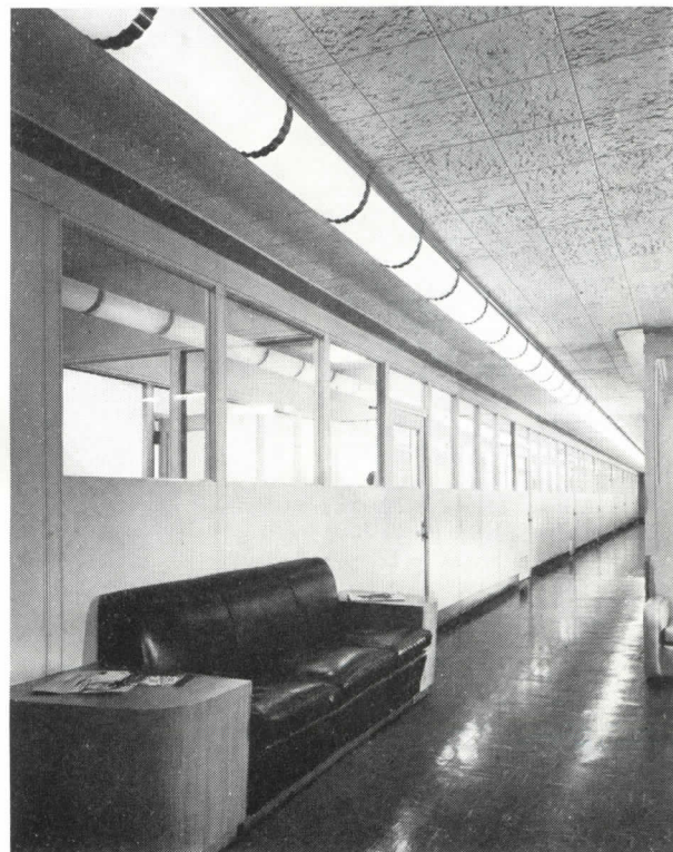
Office-building corridor, showing movable metal-and-glass partitioning.
