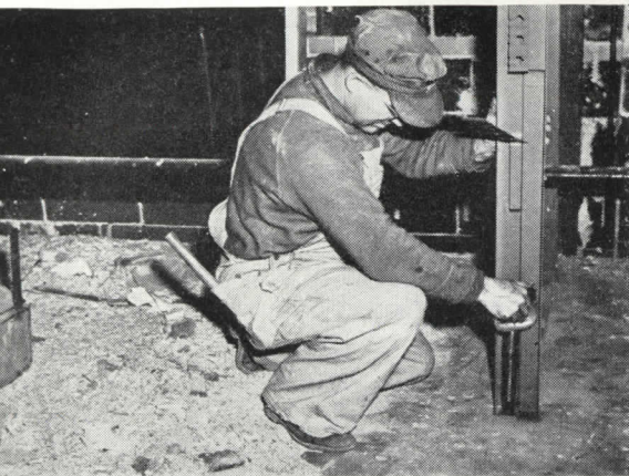
Above: workman employing powder-actuated stud-driving tool to anchor metal door frame to concrete floor. Entire operation requires only a few minutes.
