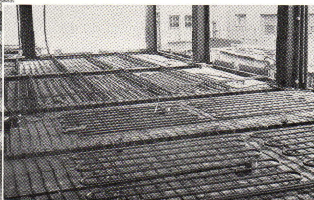
City Investing Company, builder of this structure utilized steel pipe coils in the ceilings, with some supplemental wall piping and a few floor coils. Photo shows ceiling coils viewed from floor above.
